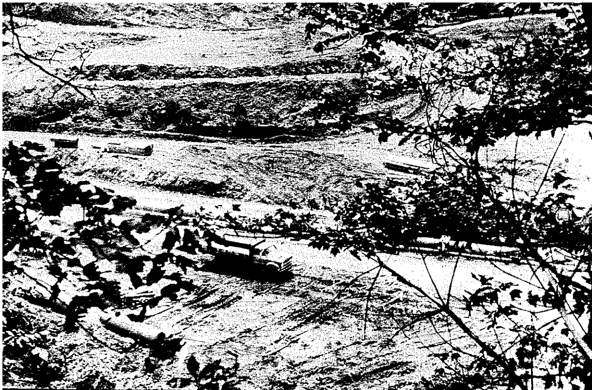
PLATE 491 Excavating for the lake at Taylor's Chapel.
