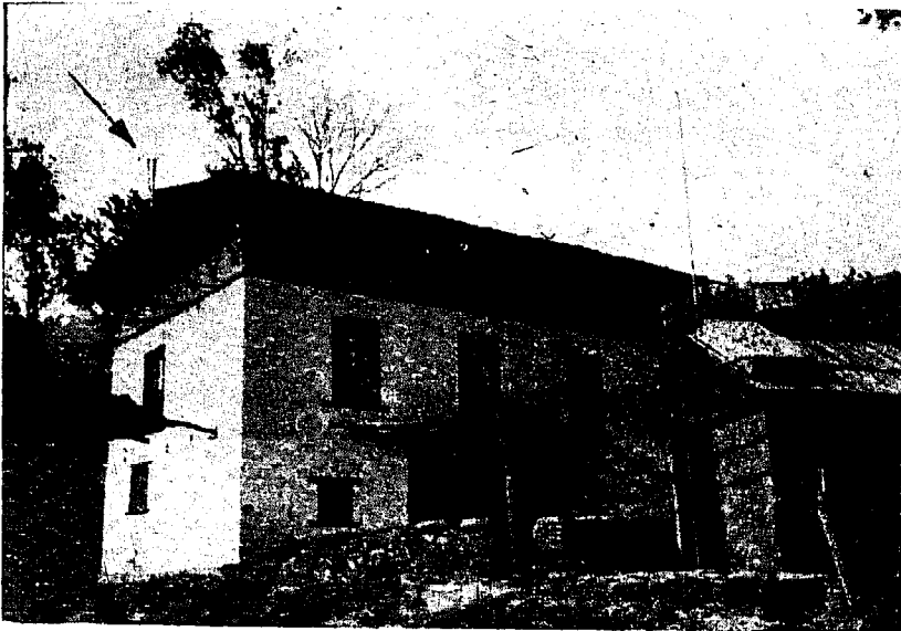
Solar powered field station: a small solar cell panel (left side, top of the house) provides electric light. A solar collector on the small house gives hot water.
