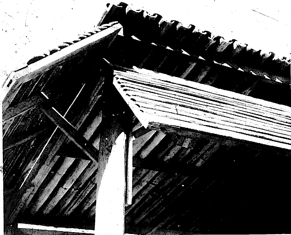
Figure XXIII. Bamboo tile roof of a hut at the Forest Research Institute, Dehra Dun, India
