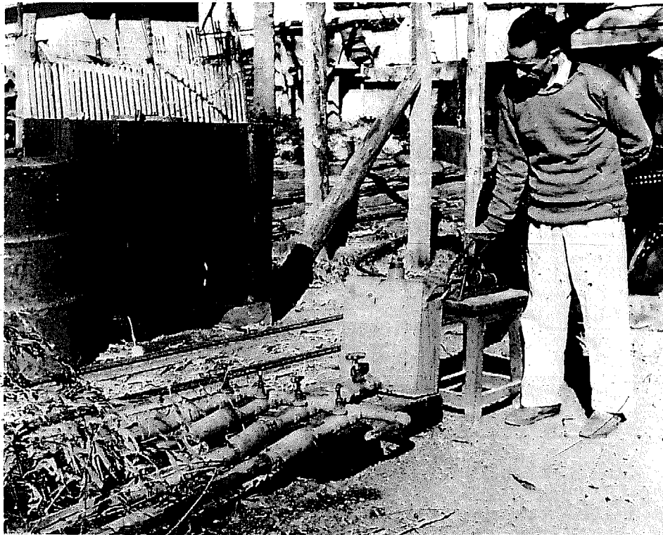
Figure XI. Modified Boucherie process for treating bamboo showing four culms connected to reservoir of preservative and hand-operated pump for applying pneumatic pressure (Forest Research Institute, Dehra Dun, India)
