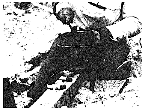
Figure 13.23 (right)—Mounting the draft-hole collar.
