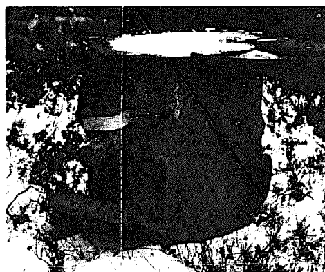
Figure 16.7 (left)—Vertical two-thirds-barrel stove, with oven. The firebox is in the upper half, the oven below. Made by Isaac Douglas.
