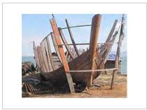
Plank on frame construction. Quy Nhon.
