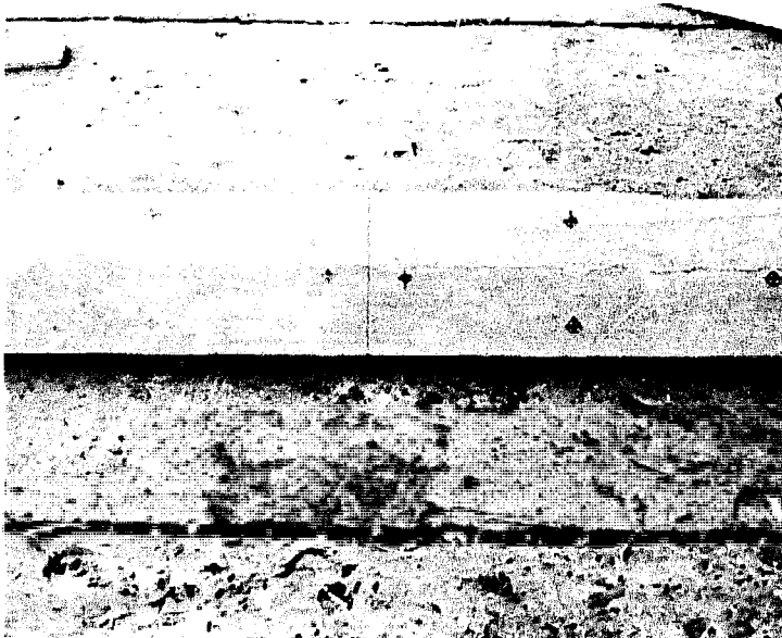
Fig.140 Marquer le centre de la cale-entretoise et pointer 8 clous Fig.140 Mark centre of the jointing plank and nail down with 8 nails
