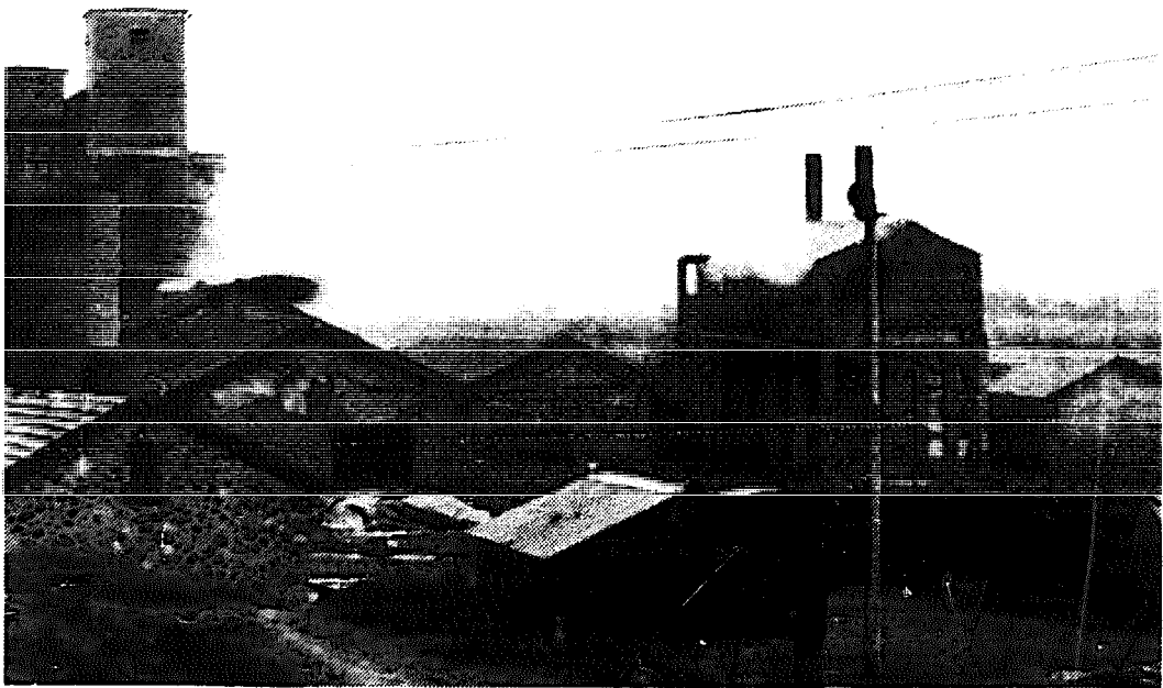
Fig 2. Small scale cement plant, China Capacity 100 tonnes/day
