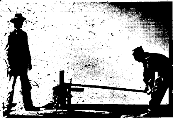
Fig. 37 (c) Maximum compaction of the block.
