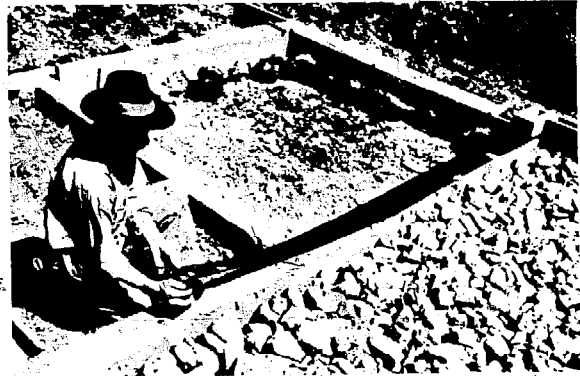
Fig. 55 Damp course of bituminous felt.
