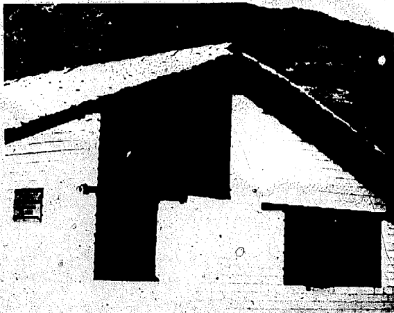
Fig. 73 Wall beam constructed directly onto the wall.
