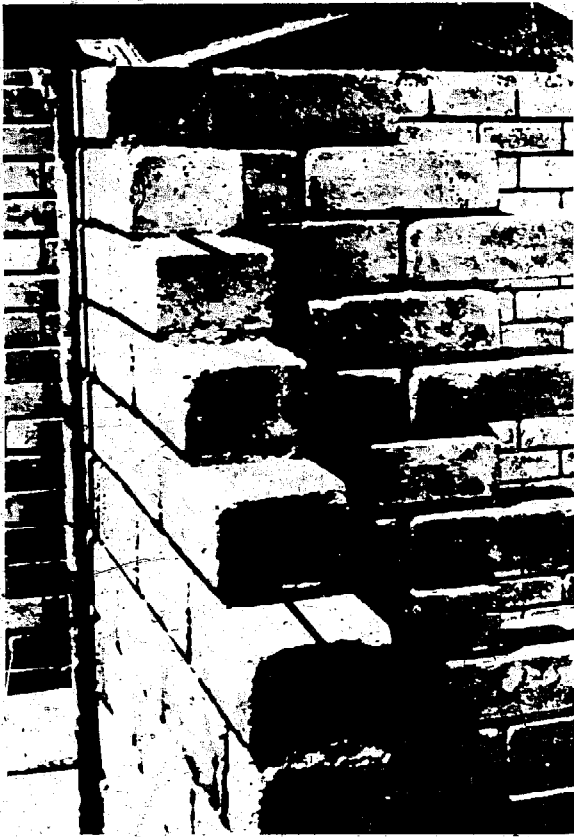
Fig. 66 Extra metal reinforcements for walls of soil-cement blocks are highly desirable in active seismic regions.
