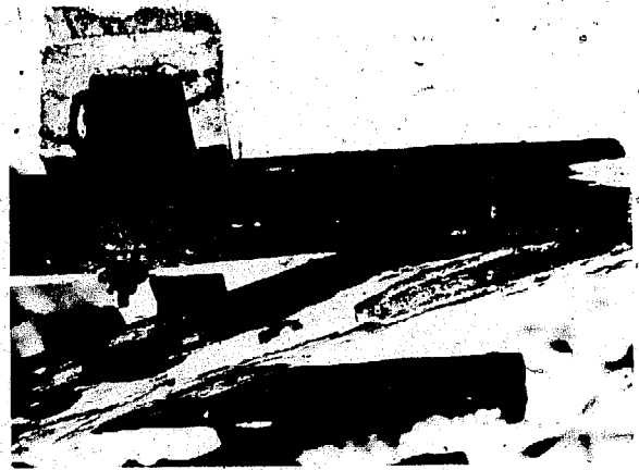
Fig. 65 (a) U-blocks used for a beam.
