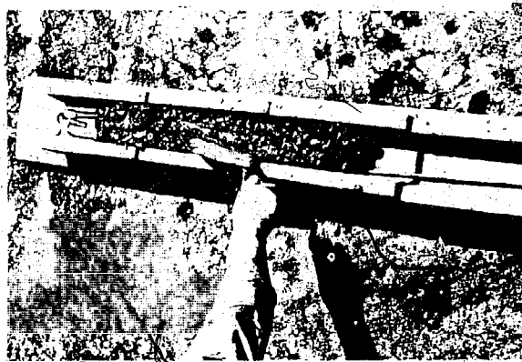
Fig. 68 Lintel prefabricated in U-blocks.
