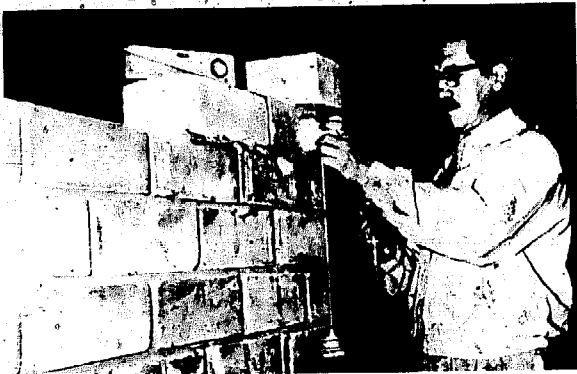
Fig. 56 Building a wall of soil-cement blocks.
