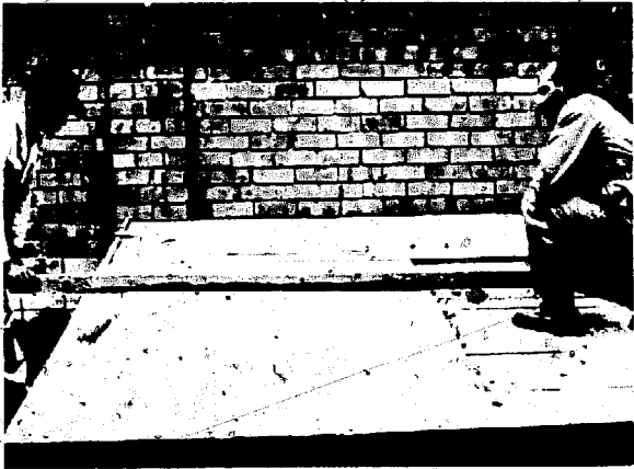
Fig. 79 Compacting the layer of soil-cement.
