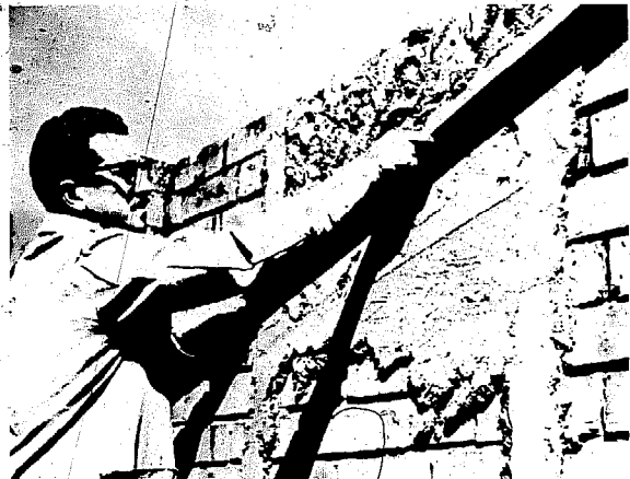
Fig. 91 Using the scraper in plastering a wall.
