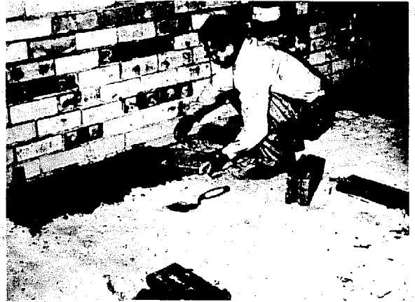
Fig. 86 Laying floor tiles.
