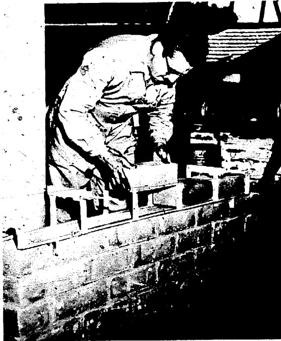
Fig. 58 Laying soil-cement blocks with a "block fitter".
