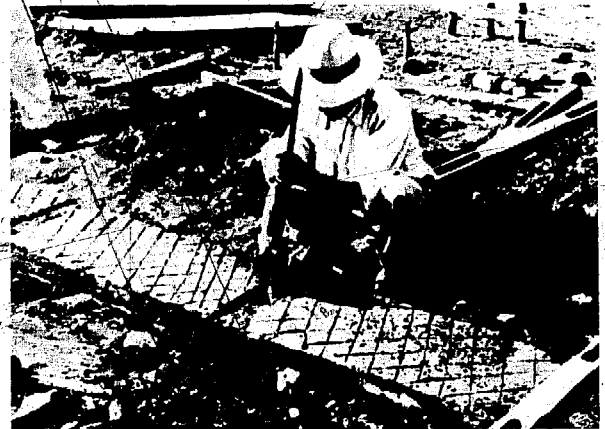
Fig. 53 Upper foundation of rammed soil-cement.
