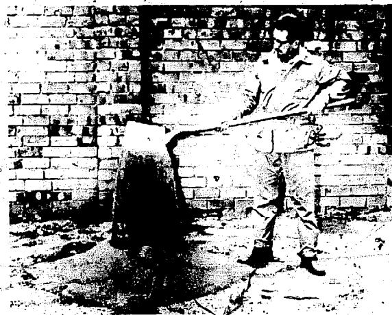
Fig. 26 Adding cement to the soil.
