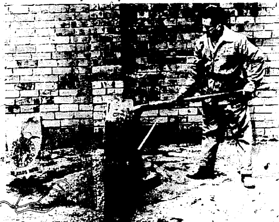
Fig. 26 (a) Mixing soil and cement.
