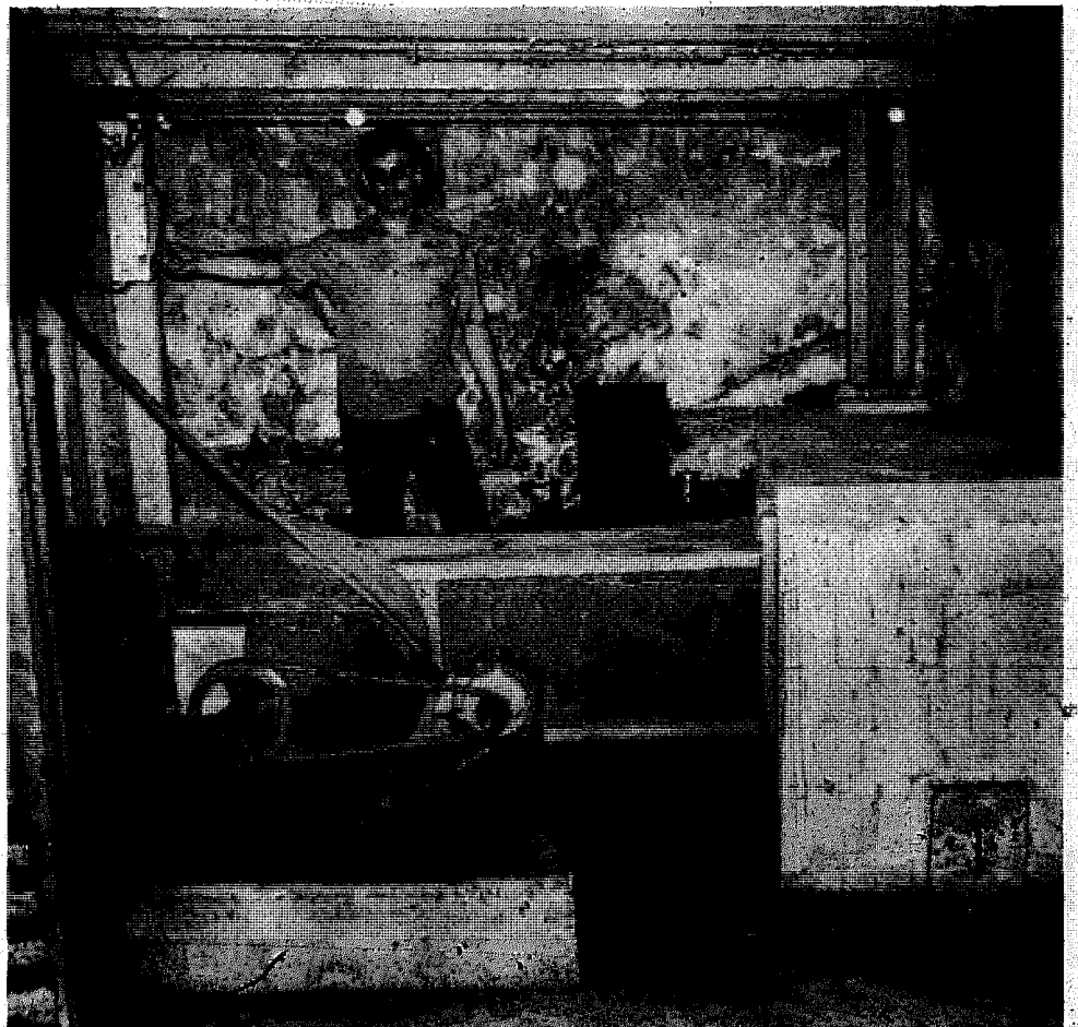
The furnace, at right, is connected to the centrifugal blower by a duct. The control switch in the upper left-hand corner should be located near the control for the rice hulls.
