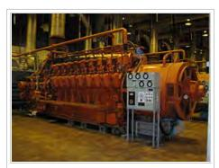
Big Diesel generator used for backup power
