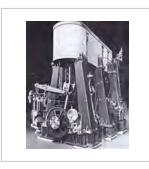
140-ton – also described as 135-ton – vertical tripleexpansion engine of the type used to power World War II Liberty ships, assembled for testing prior to delivery. The engine is 21 feet (6.4 meters) long and 19 feet (5.8 meters) tall and was designed to operate at 76 rpm and propel a Liberty ship at about 11 knots (12.7 mph; 20.4 km/h).
