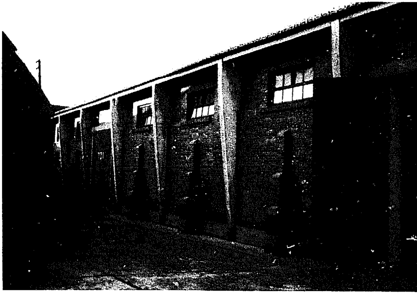
Photo 49 - Warehouse for bagged grain. Portal frames at cc 4 m. Buttresses between portal frames. (Seventh Depot, Shanghai)
