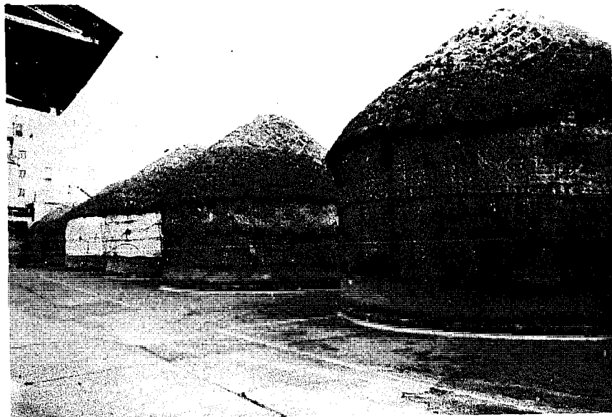
Photo 63 - Outdoor bulk storage for 150 tons of paddy. Walls built from bags filled with paddy, interior space filled with bulk paddy. The top cone is shaped by straw piled on top of the rice, then thatched and fixed with a rope net. (Xinqiao Grain Purchasing and Supply Station, Songjiang County)
