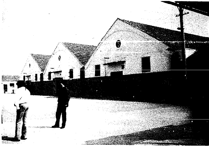
Photo 45 - Concrete dome-roofed warehouse with tile roof. Three bays, each 16 x 20 m. Built 1959. Total holding capacity 1 500 tons paddy. (Bacon Depot)
