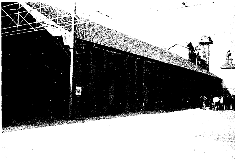
Photo 40 - Bulk grain warehouse, two sections, 20 x 24.5 m each. Type "51". (First Depot, Wuxi)
