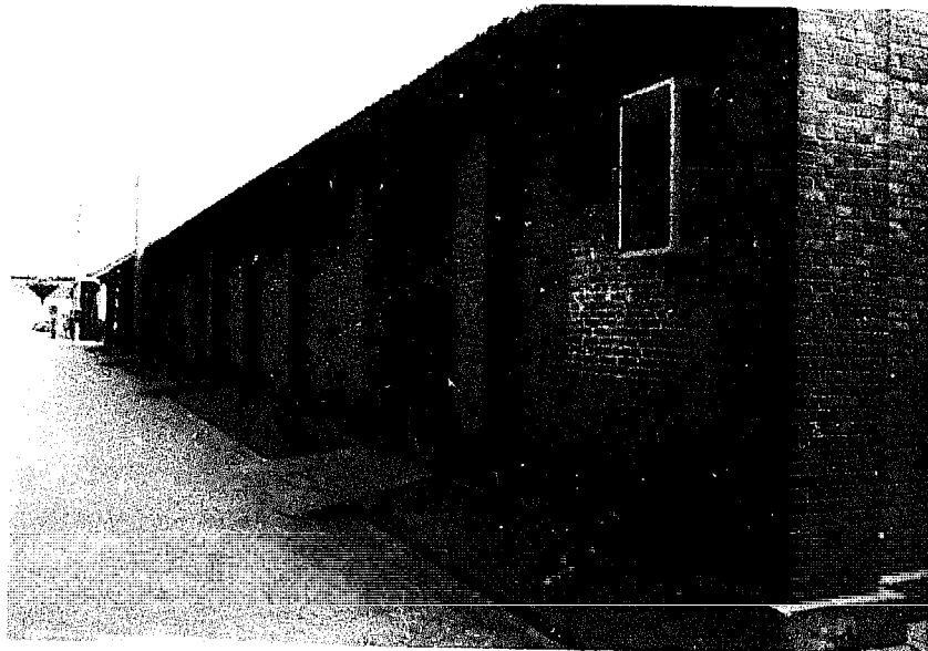
Photo 15 - Ventilation openings controlled by electric motor (Baoan Depot)
