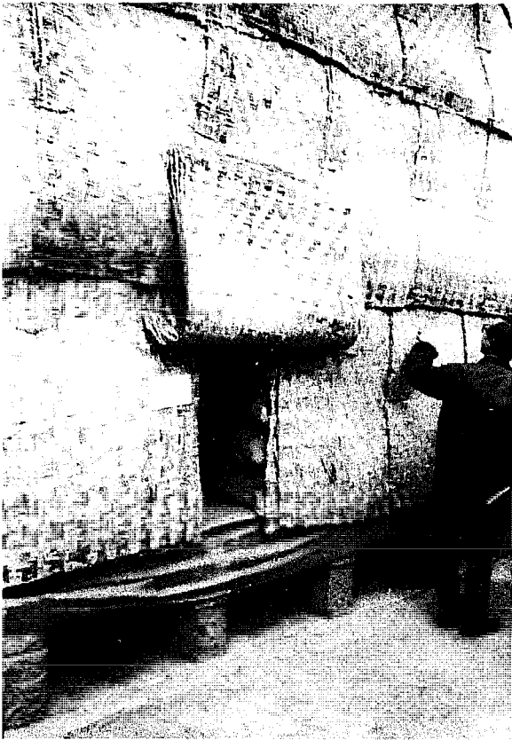
Photo 60 - Outdoor bag stack with ventilation opening 50 x 180 cm. Wall cover is double layer of reed sheets, 128 x 164 cm each. Under the stack, polyethylene sheets and reed mats on wooden platform.
