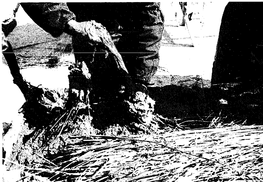
Photo 25 - When straw bundles are thoroughly covered with clay mud, excess mud is removed. (Niou Pao Tun Depot)
