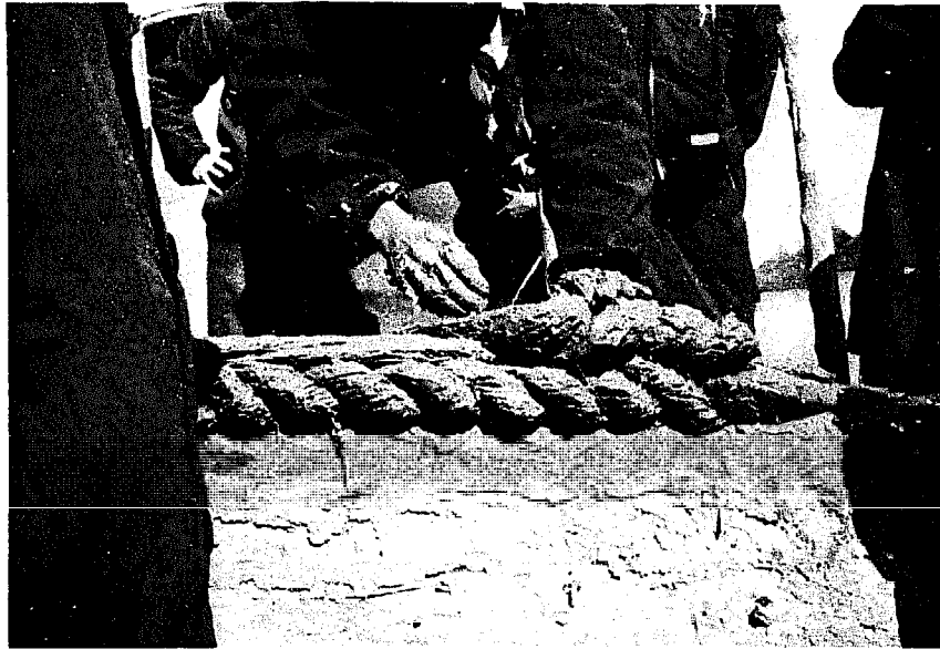
Photo 32 - Construction of eaves. The first layer has been placed and second layer is being started, with the clay/straw bundles turning in the opposite direction. (Niou Pao Tun Depot)
