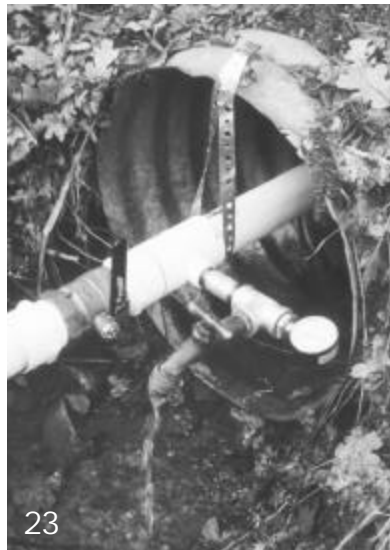
23. The drain valve, inline ball valve, and pressure gauge are clustered together about 10 feet from the hydro unit.
