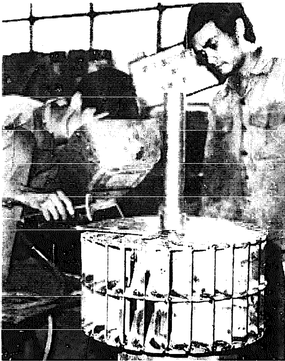
Fig. 26: Welding of Rotor T1
