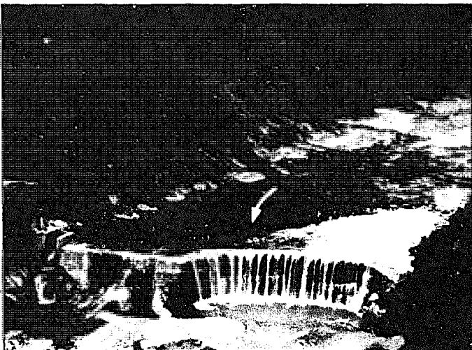
Fig. 5.28. A temporary diversion weir across the stream is used to divert water toward an underground intake at the left. This dam is used only to increase head; it does not form a reservoir to store water.
