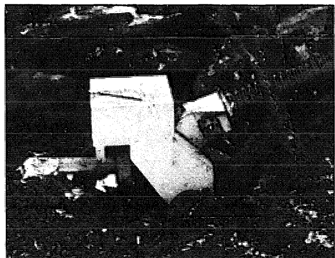
Fig. 5.24. At this site which has been in operation since 1975, a simple metal box hinged on one side and a belt guard protect the turbo-generating equipment from the elements. See Fig. 6.9 for a view of the unit with the cover removed.
