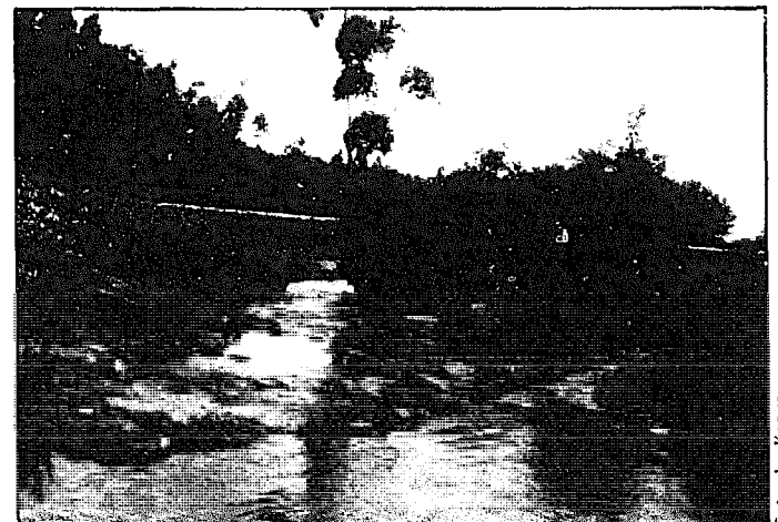
Fig. 5.26. A simple weir of loose stones diverts water to a small turbine-driven mill.
