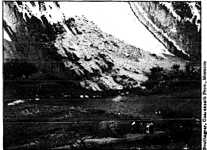
Fig. 5.44. Intake to a traditional irrigation canal. Despite the fact that the beginning of the canal is oriented nearly parallel to the stream, a rock outcropping deflects water toward the right bank during the river's high stage. The temporary weir would also wash away.
