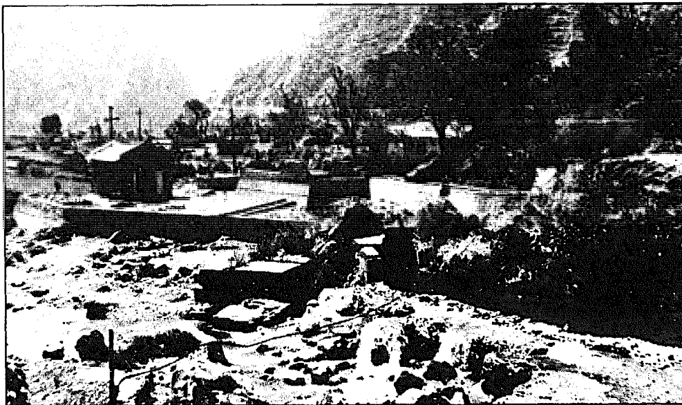
Fig. 4.13. At this site, irrigation water was initially diverted through an intake at the center of the left photograph. The powerhouse visible on the left was later constructed, and water for power generation is diverted into a power canal from the same stream somewhat upstream of
