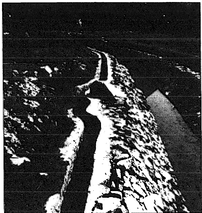
Fig. 5.76. The portion of this canal where soil is not very porous is lined with stones. The small uphill canal serves as a settling area for uphill runoff and is paved to facilitate cleaning. No drainage around the canal has been incorporated.
