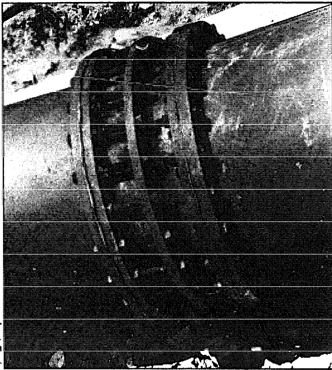
Fig. 5.134. A sliding-type expansion joint.
