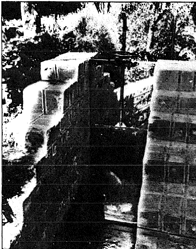
Fig. 5.175. Steel sliding gate operated by a handwheel.
