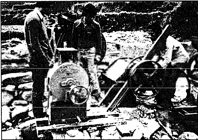
Fig. 10.29. The new turbines are mounted above the mill floor on a common mounting frame, which is eventually set in concrete. Here the installation team is shown using a string to align the pulleys.
