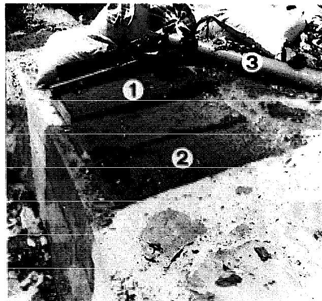
Fig. 20: Tirolian weir type intake . 1 Trash rack 2 Perforated plate cover over trash rack 3 Overflow from drinking water supply (PVC pipe, outside dia. 90 mm)
