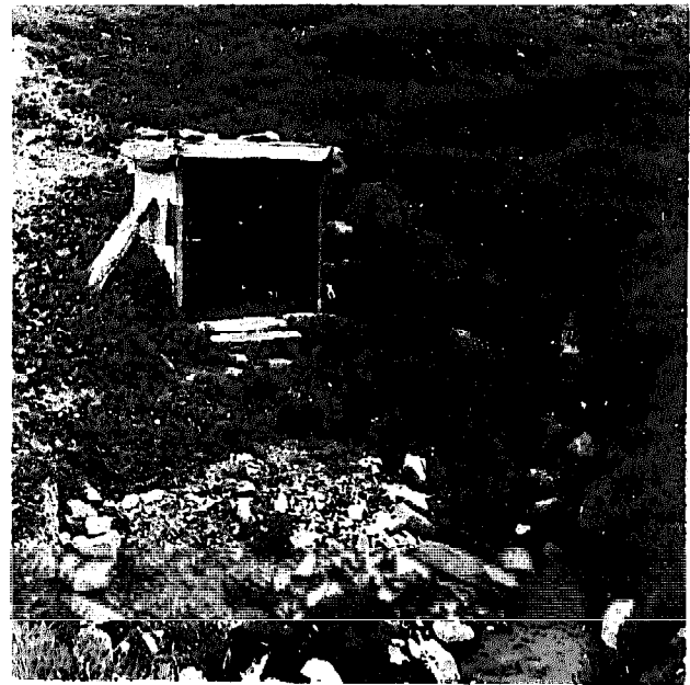
Fig. 6: Machine house: By covering it with earth and planting the appearance could be improved.
