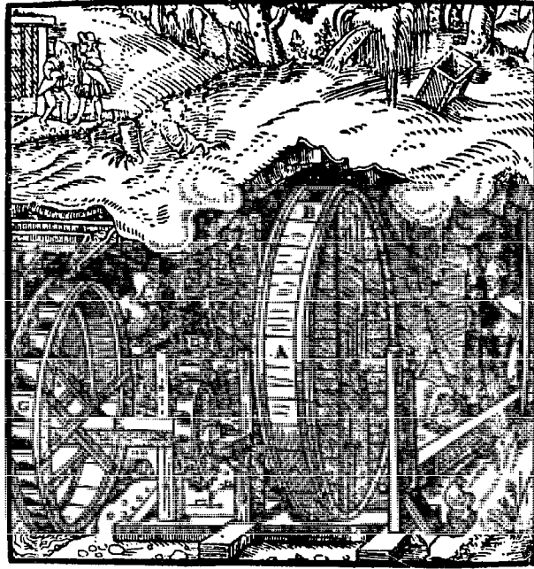
fig. 43: Ventilating air pump.
