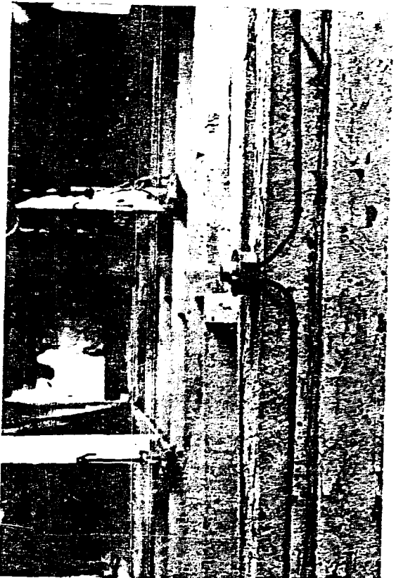
Figure 17. NON-METALLIC SHEATHED CABLE IN A DAIRY BARN.
