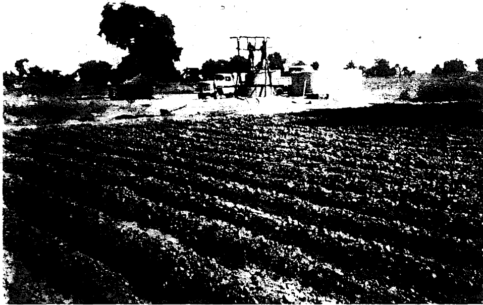
Large diameter self-help well equipped with animal-drawn skin bucket and small reservoir for irrigating vegetable crops
