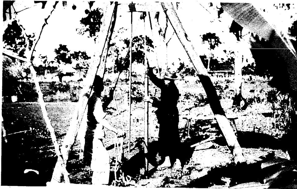
Fig. 19 Bailing well with 6 cm diameter bailer
