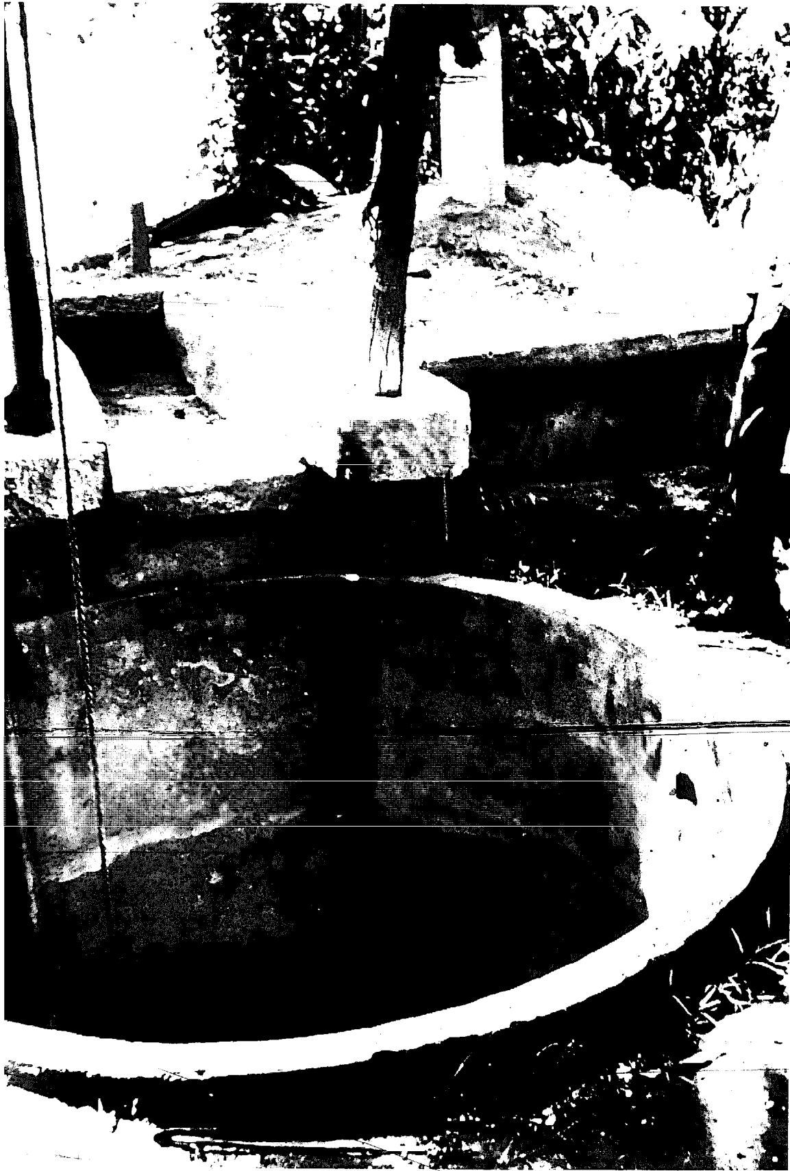
6 diameter well equipped with stone channel to irrigation system into which skin buckets are emptied
