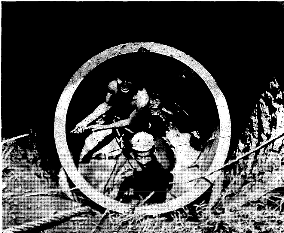
Fig. 45 Precast concrete caissons being set into a well excavated to the water table without lining
