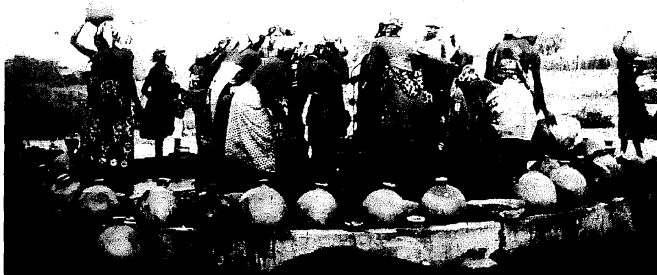
Large diameter village self-help well. (Note rim around platform to divert spilled water to animal watering trough.)
