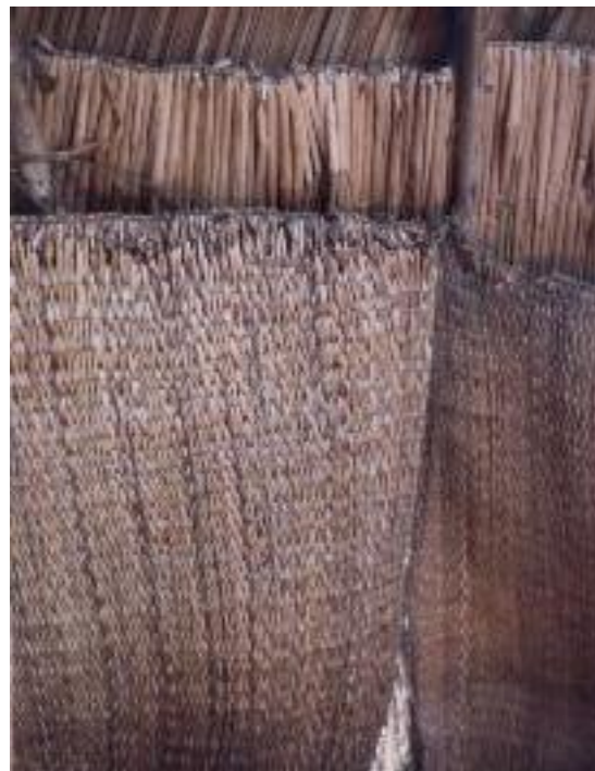
WOVEN INTERIOR MATS ON BOTTOM WITH SEWN EXTERIOR MATS SHOWING BEHIND ON
