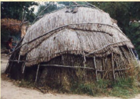
A completed family wigwam at Plimoth Plantation showing bark sheets on the bottom, and cattail mats covering the top.
