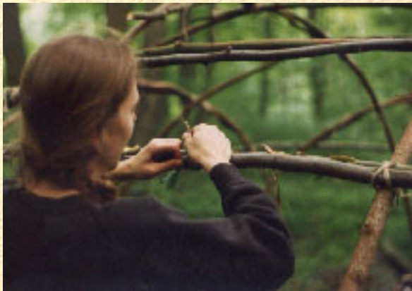
Me, lashing the hoops onto the wigwam poles, which gives the structure added support.
