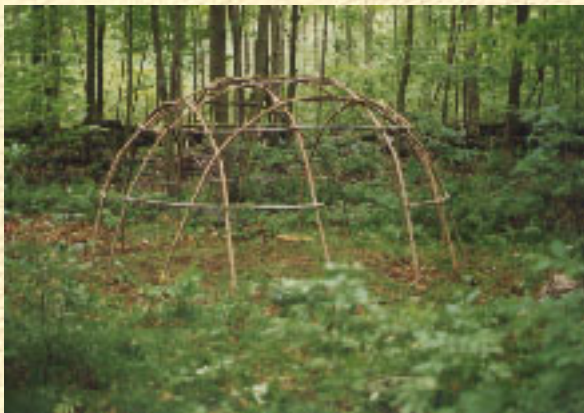
The completed sapling frame of my wigwam in the northeastern connecticut woods. The poles are made of sassafrass, the hoops are made of sweet birch.
