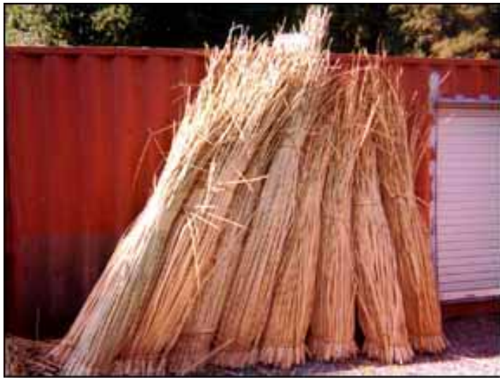
Eight 8-foot tule mats ready to be tied onto the house frame.
