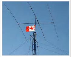
The top of a tower supporting a Yagi-Uda antenna and several wire antennas
