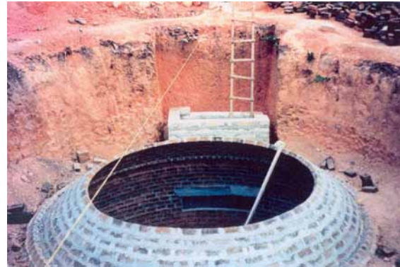
Fig. 9: Biolatrine for 2x3 toilets, 200 people in Kumasi, Ghana (under constr.) front: digester, rear: influent shaft (Source: [3])
