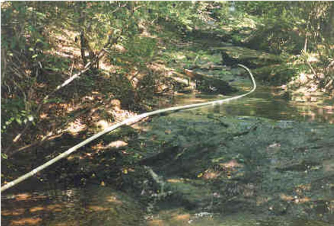
Figure 2. The 1-1/4 inch Schedule 40 PVC drive pipe supplying the ram pump. Note the curves in the pipe due to the geometry of the stream channel. The pump worked quite well despite the lack of straightness of the pipe.
