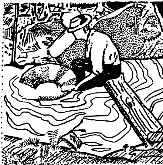
Fig. 8 Concentration of material with a batea
