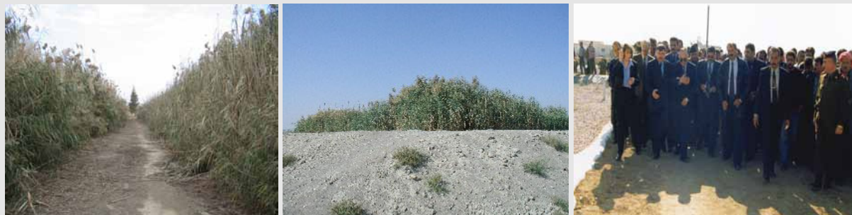
Figure 28: Constructed wetland reed beds (left); sludge reed bed (middle); official inauguration of the pilot project (right). (Mohamed)
