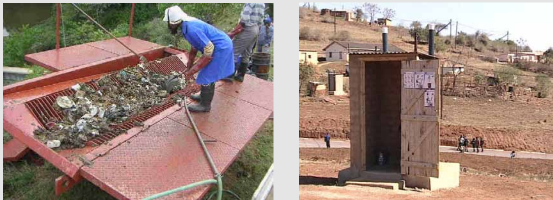
Figure 1: Emptying conventional pit toilets required special equipment (left picture) and turned out to be extremely costly - often exceeding 1000 Rand per pit. The urine diversion dehydration toilet (right picture) was selected by the communities as preferred solution after extensive awareness raising measures (Macleod 2005).
