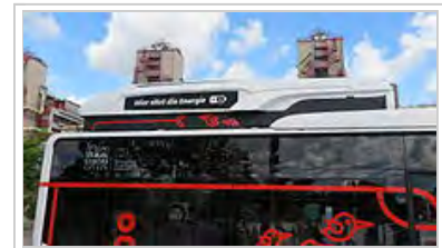
Battery pack on the roof of a battery electric bus
