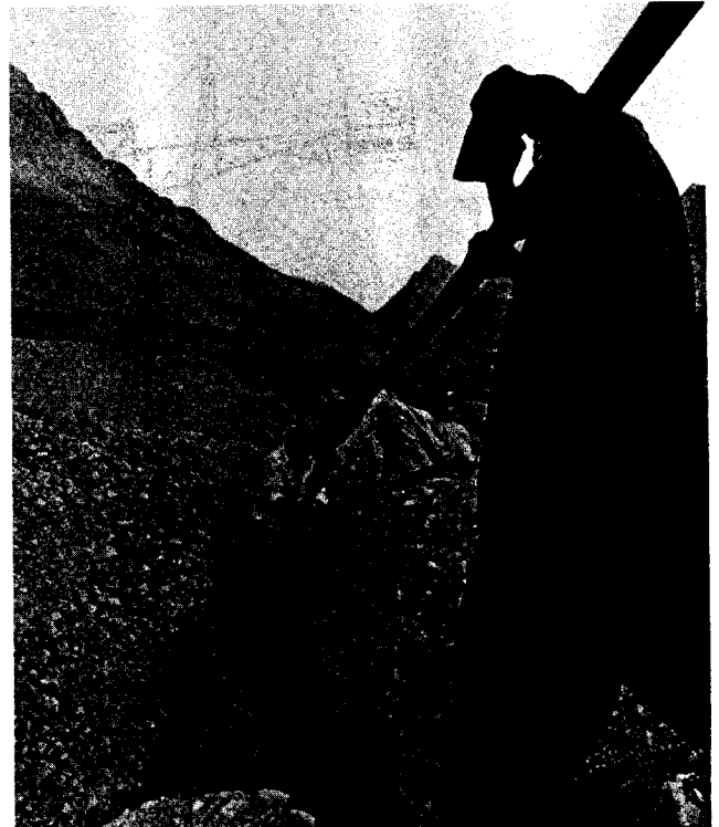
Plate 51 Laying the pipeline
