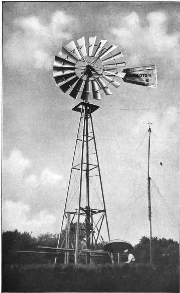
VIEW OF MILL NO. 44—16-FOOT AERMOTOR.
