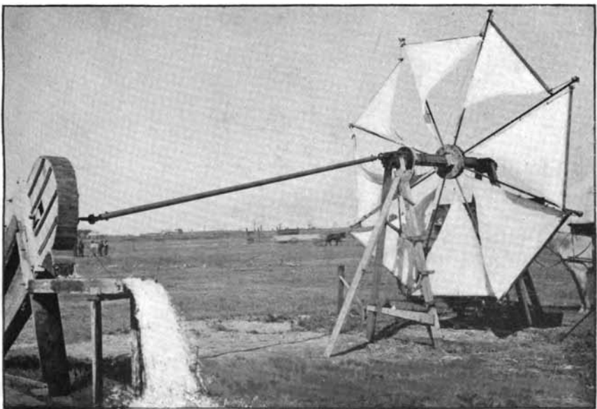
B. VIEW OF DEFENDER MILL AND PUMP KNOWN AS "WATER ELEVATOR."
