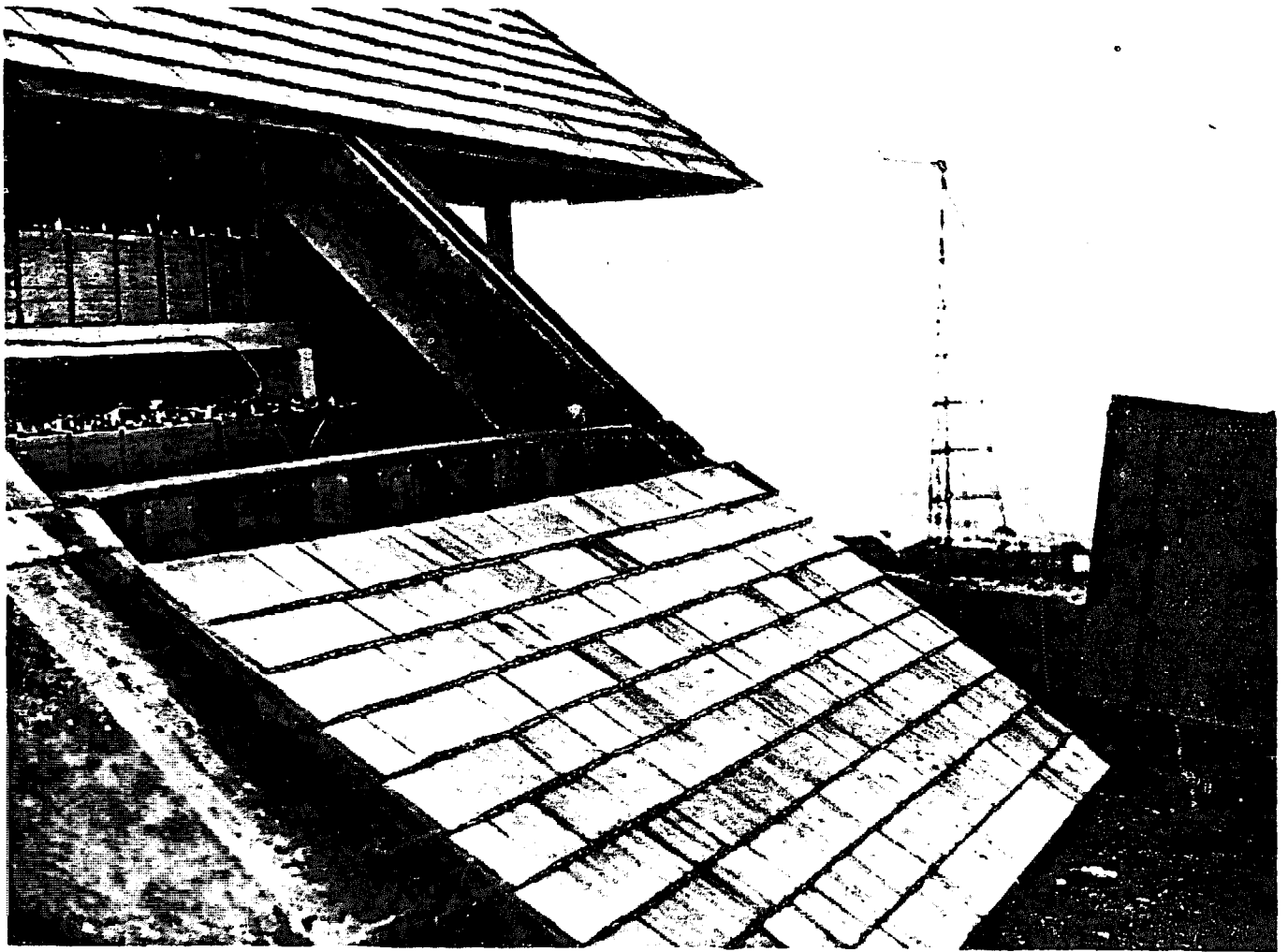
FIGURE A2-9: Battery bank installation.
