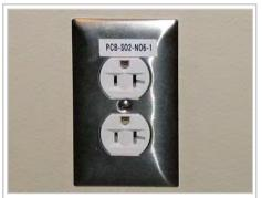
5-20RA (Canada) or 5-20R (USA) T-slot socket mounted with the earth hole up. The neutral connection is the wider T-shaped slot on the right.
