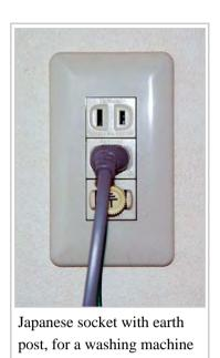
stricter dimensional requirements for the plug housing, different marking requirements, and mandatory testing and approval by METI or JIS.<sup>[77]</sup>
