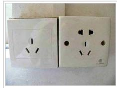
Chinese 3-pin socket and compound socket which also accepts NEMA and Europlug (right), and a less common 16 A version (left)
