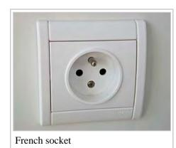
The CEE 7/5 socket and CEE 7/6 plug are defined in French standard *NF C 61-314 "Plugs and socket-outlets for household and similar purposes"* (which also includes CEE 7/7, 7/16 and 7/17 plugs) The socket has a predominantly circular recess which is 15 mm (0.591 in) deep with two symmetrical round apertures
