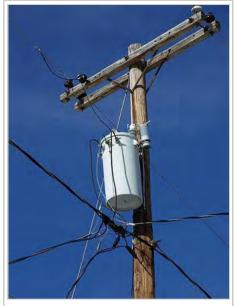
US single-phase residential power distribution transformer, showing the two insulated "Line" conductors and the bare "Neutral" conductor (derived from the earthed center-tap of the transformer). The distribution supporting centenaries are also shown.
