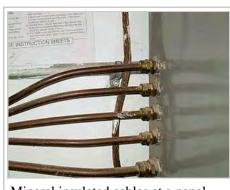
Mineral insulated cables at a panel board
