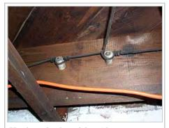
Knob-and-tube wiring (the orange cable is an unrelated extension cord)
