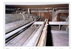
Electrical conduit risers, seen inside fire-resistance rated shaft, as seen entering bottom of a firestop. The firestop is made of firestop mortar on top, rockwool on the bottom.
