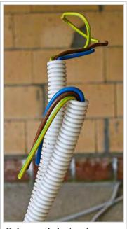
Colour-coded wires in a flexible plastic electrical conduit found commonly in modern European houses
