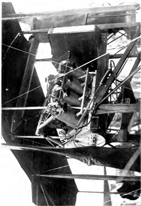
PLATE XXII. Engine and Propeller of Curtiss Aeroplane.
