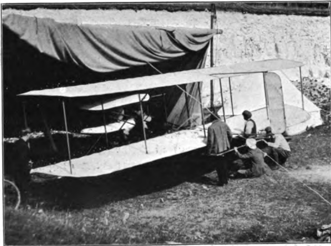
FIG. 83.—Special Temporary Hangar for Biplane Glider. This Machine has a Span of 33 ft.
