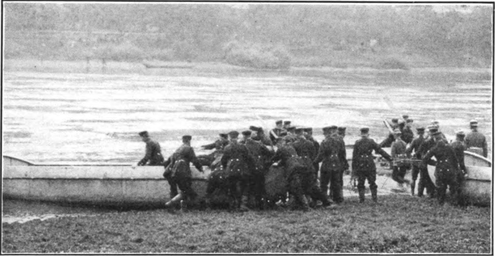
Floating the pontoons
