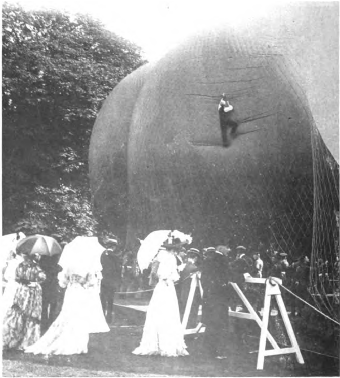
CLIMBING THE NET TO MAKE A REPAIR.
