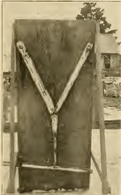
REAR VIEW, DEVICE FOR HOLDING FRAMES ON THE SQUARE FOR NAILING
