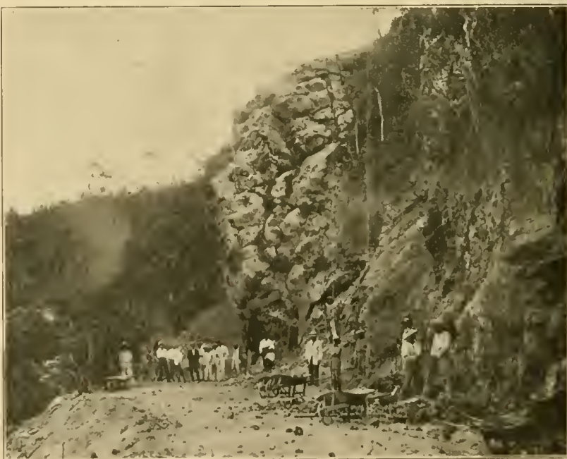
BUILDING A MOUNTAIN ROAD IN PORTO RICO
