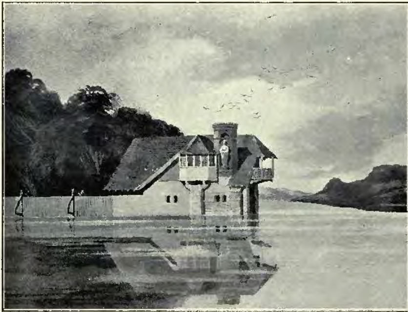
Rudyard Lake Boathouse , THE LATE LARNER SUGDEN, F.R.I.B.A., Architect.
