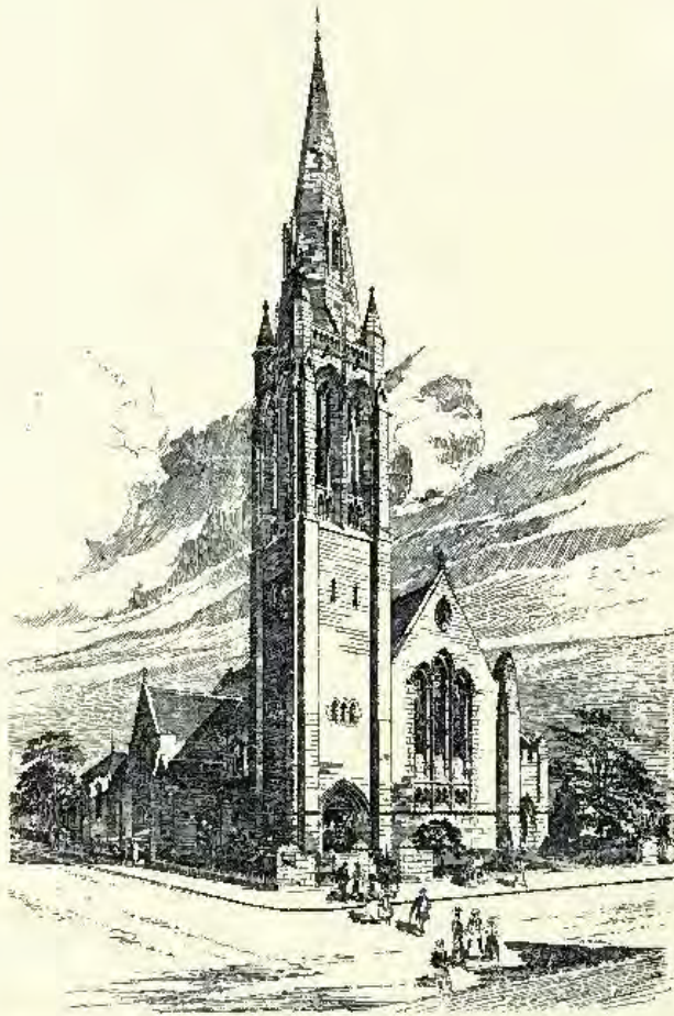
544. Beechgrove U. F. Church, Aberdeen, BROWN AND WATT, Architects.
