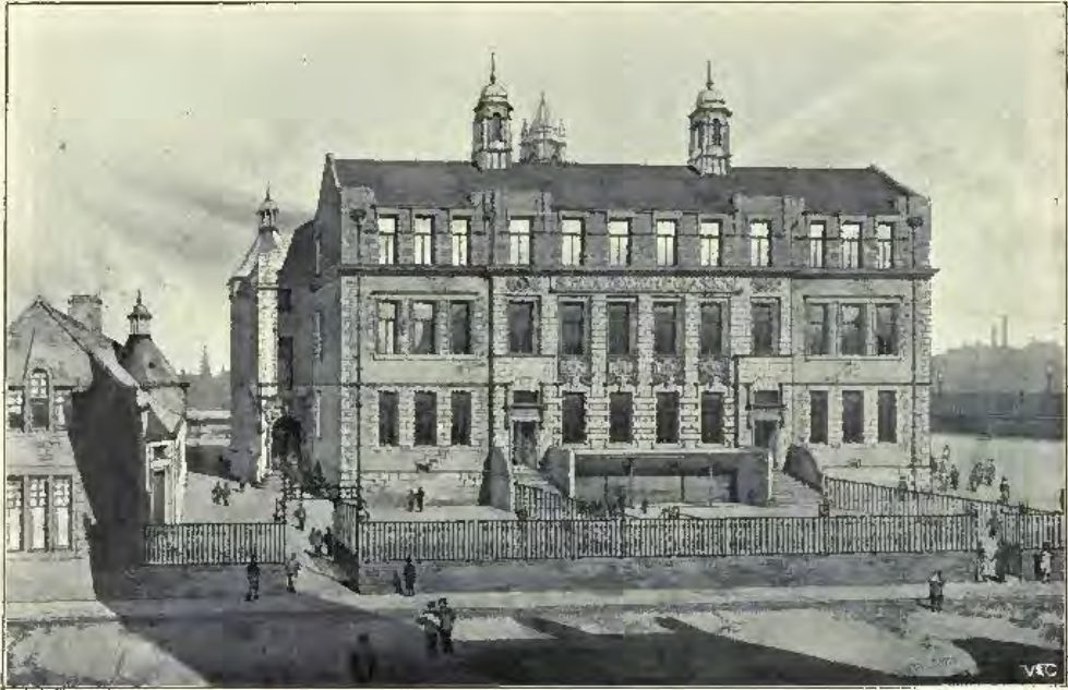
531. Golf Hill School, Dennistoun, for the School Board of Glasgow, ALEXANDER N. PATERSON, M.A., Architect.
