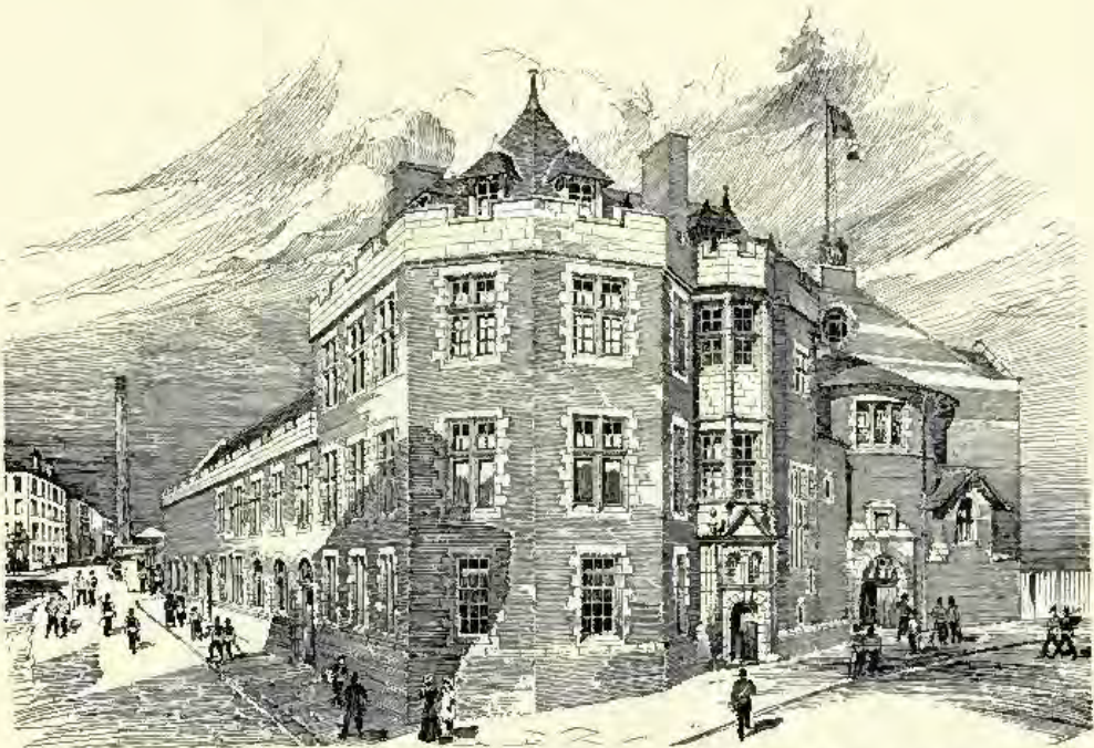
526. Headquarters and Drill Hall, Yorkhill, for 2na V.B.H.I., WILLIAM II. M'NAB, Architect.
