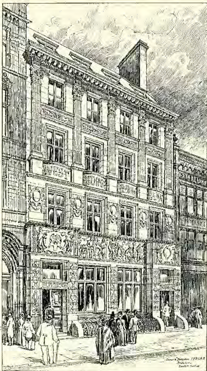
1548. West Riding Union Bank, Park Row, Leeds, OLIVER AND DODGSHUN, Architects.
