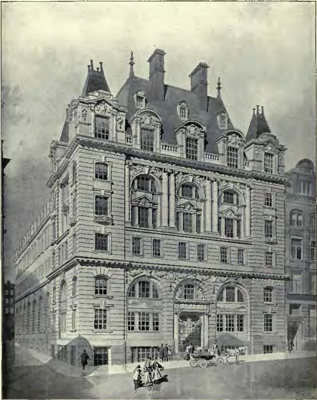
1385. Messrs. Elder, Dempster & Co.'s New Head Offices, Liverpool, BRIGGS AND WOLSTENHOLME, F. B. HOBBS AND ARNOLD THORNELY, Architects.
