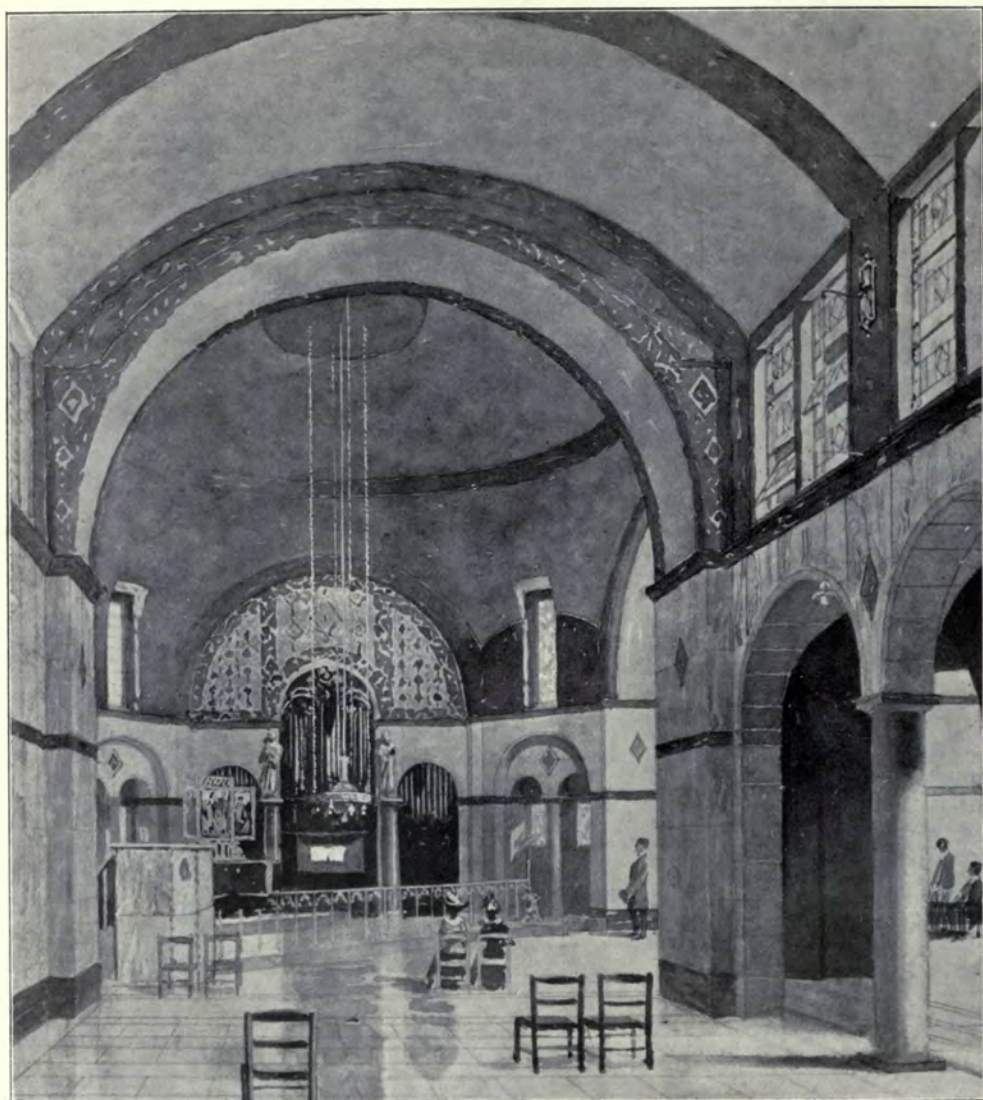
1534. Open Air Chapel, King Edward VII. Sanatorium, H. PERCY ADAMS, Architect.
