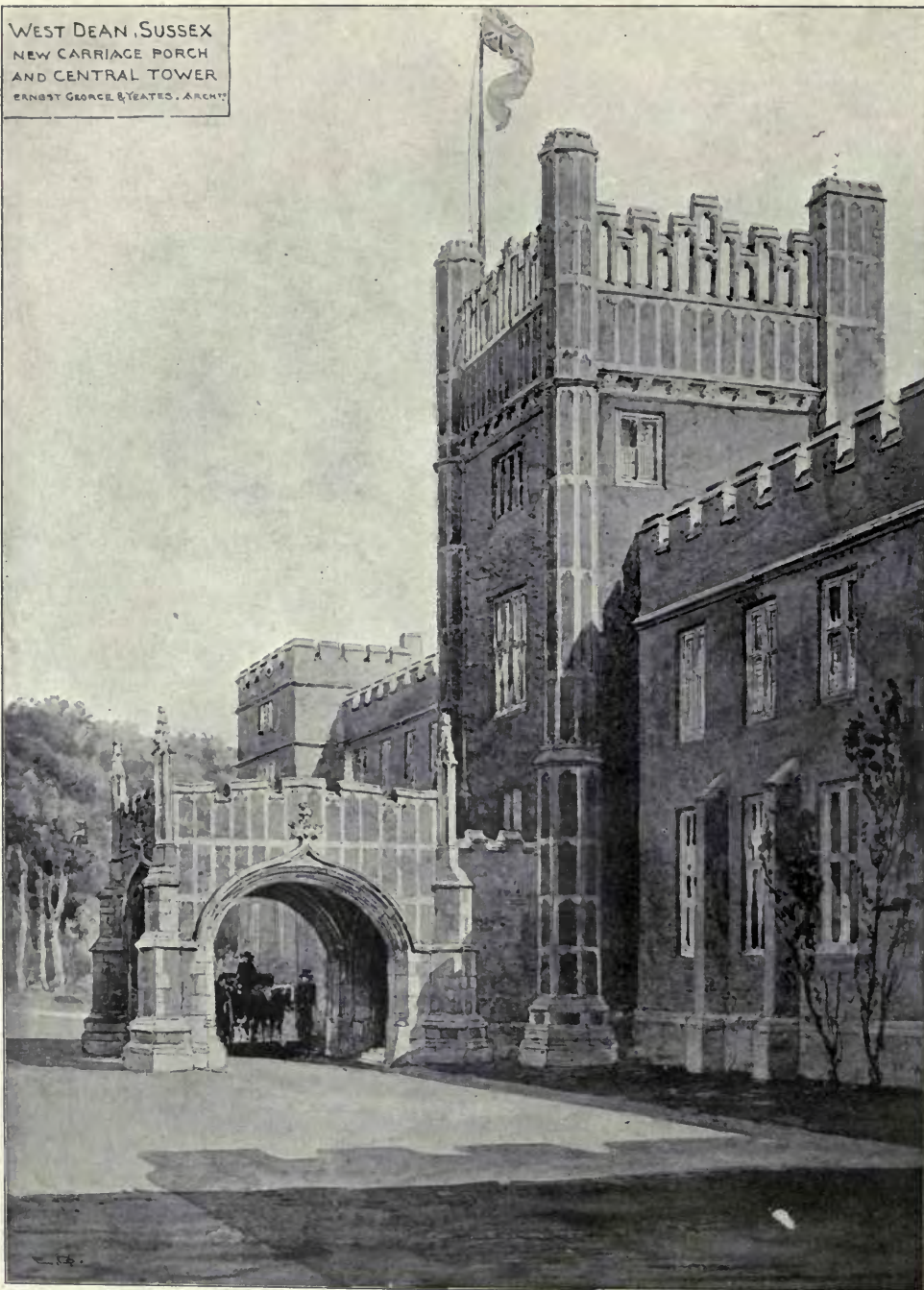
1468. New Carriage Porch and Central Tower, West Dean, Sussex, ERNEST GEORGE AND YEATES, Architects. Metal Casements and Leaded Glazing: R. E. Pearse and Co., Ltd., 181, Upper Kennington Lane, London, S.E.
