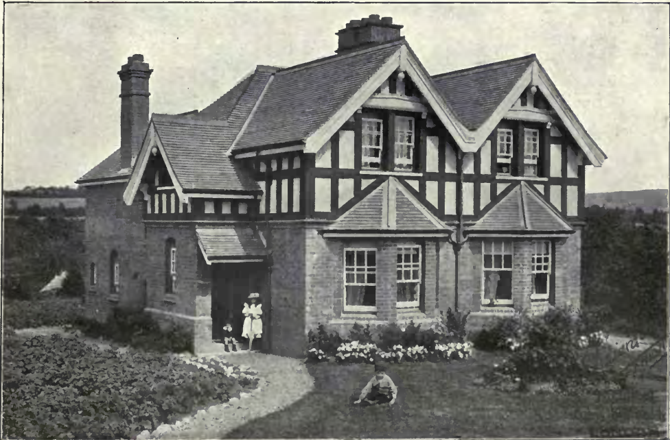
Cottages, "Southerton," Ottery St. Mary, Devon, T. E. LIDIARD JAMES, Architect. (For Plans, see p. 112.)
