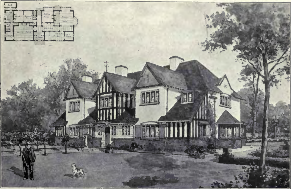
The Old Orchard House, Farnham Royal, MELVILLE S. WARD, Architect. (For Plans, see p. 109.) General Contractor: W. J. Page, Station Road, Northwood, Middlesex.
