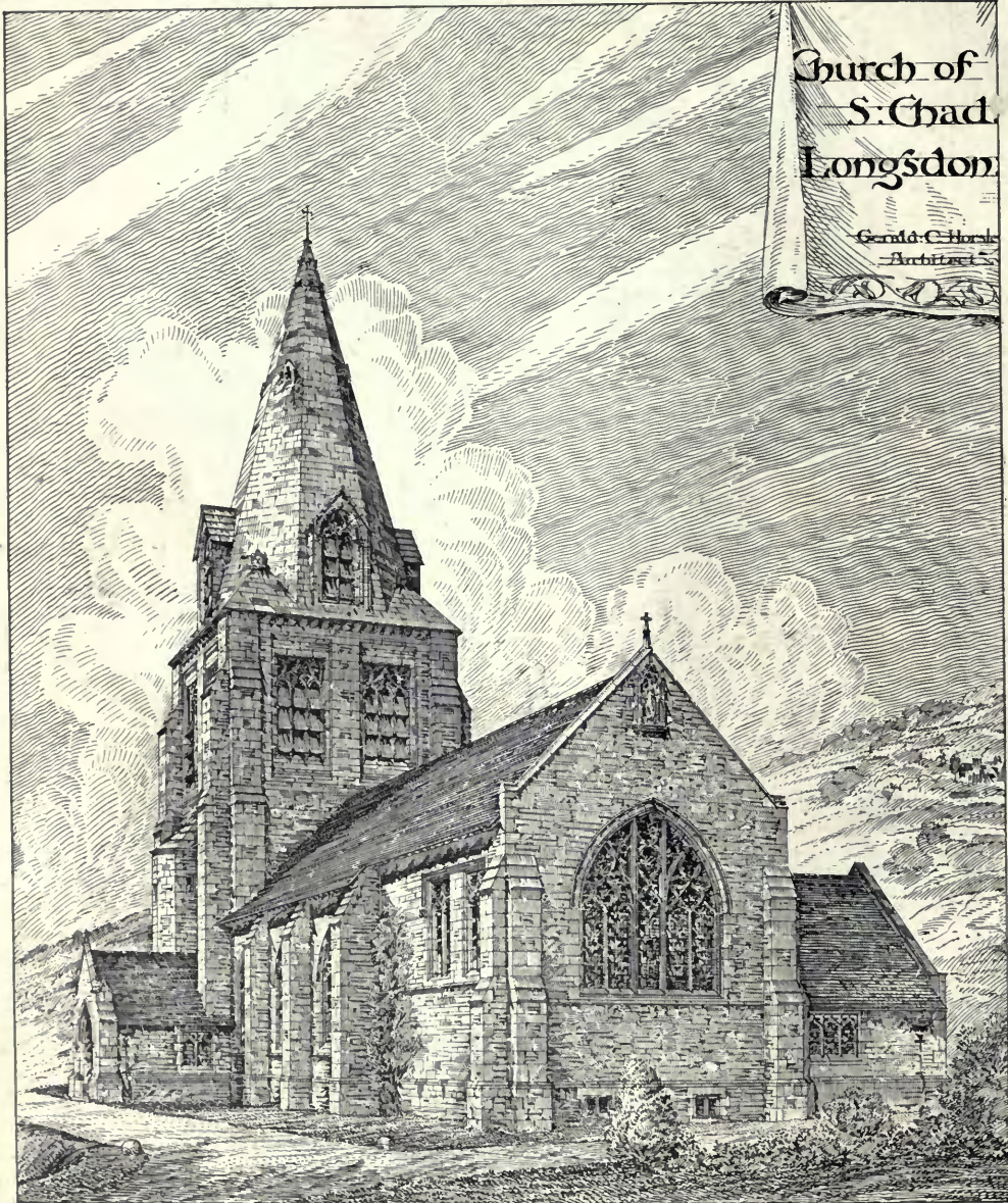
1567. Church of St. Chad, Longsdon, Staffs , GERALD C. HORSLEY, Architect. General Contractors: Thos. and Henry Grace, Broad Street, Leek, Staffordshire.
