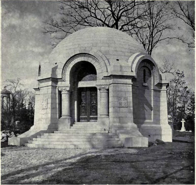
John D. Archbold Mausoleum, Sleepy Hollow Cemetery, Tarrytown, N. Y., MORRIS, BUTLER AND RODMAN, Architects.
