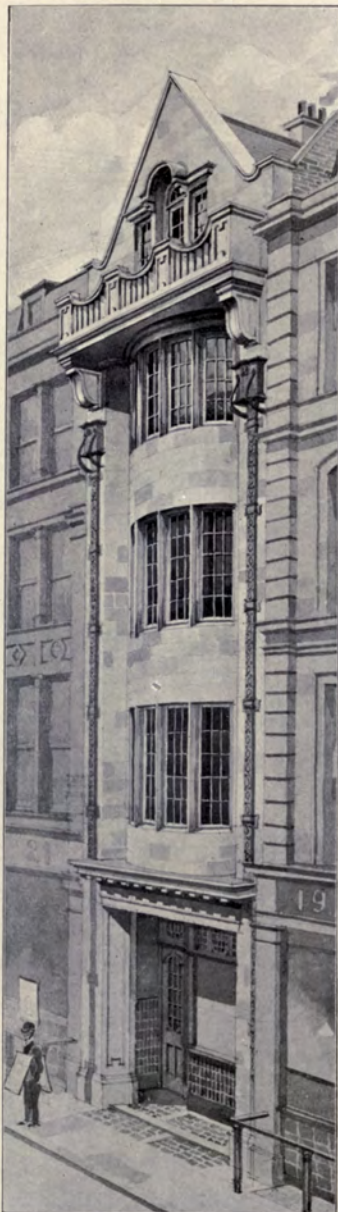
1474. Premises, Warwick Street, Regent Street, W., JOHN N. R. VINING, Architect. General Contractors, Bywaters and Sons, 10 Kingly St., W. Iron Casements, Henry Hope and Son, Ltd., 55 Lionel Street, Birmingham.
