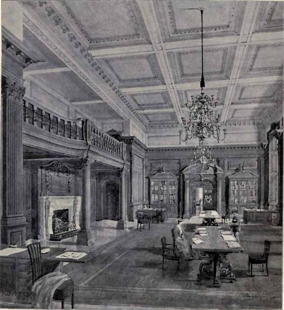
1542. New Buildings, 160, Wardour Street: Interior , FRANK L. PEARSON, Architect. Contractors, H. H. Martyn and Co., Ltd., Cheltenham.
