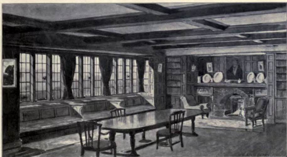
1635. Dining-room, House at Hailsham, W. H. ATKIN BERRY, Architect. Contractor, P. Hide, Hailsham.
