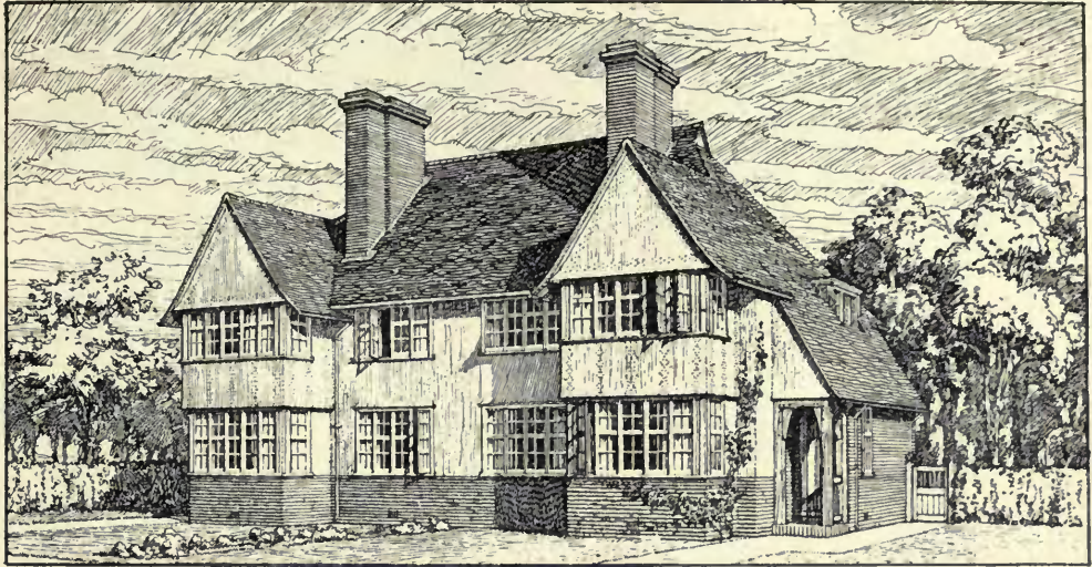
Houses at Hampstead, Willifield Way, GEOFFRY LUCAS, Architect. (For Plans, see p. 139.) Contractors: William Moss and Sons, Ltd., Loughborough, Leicestershire.
