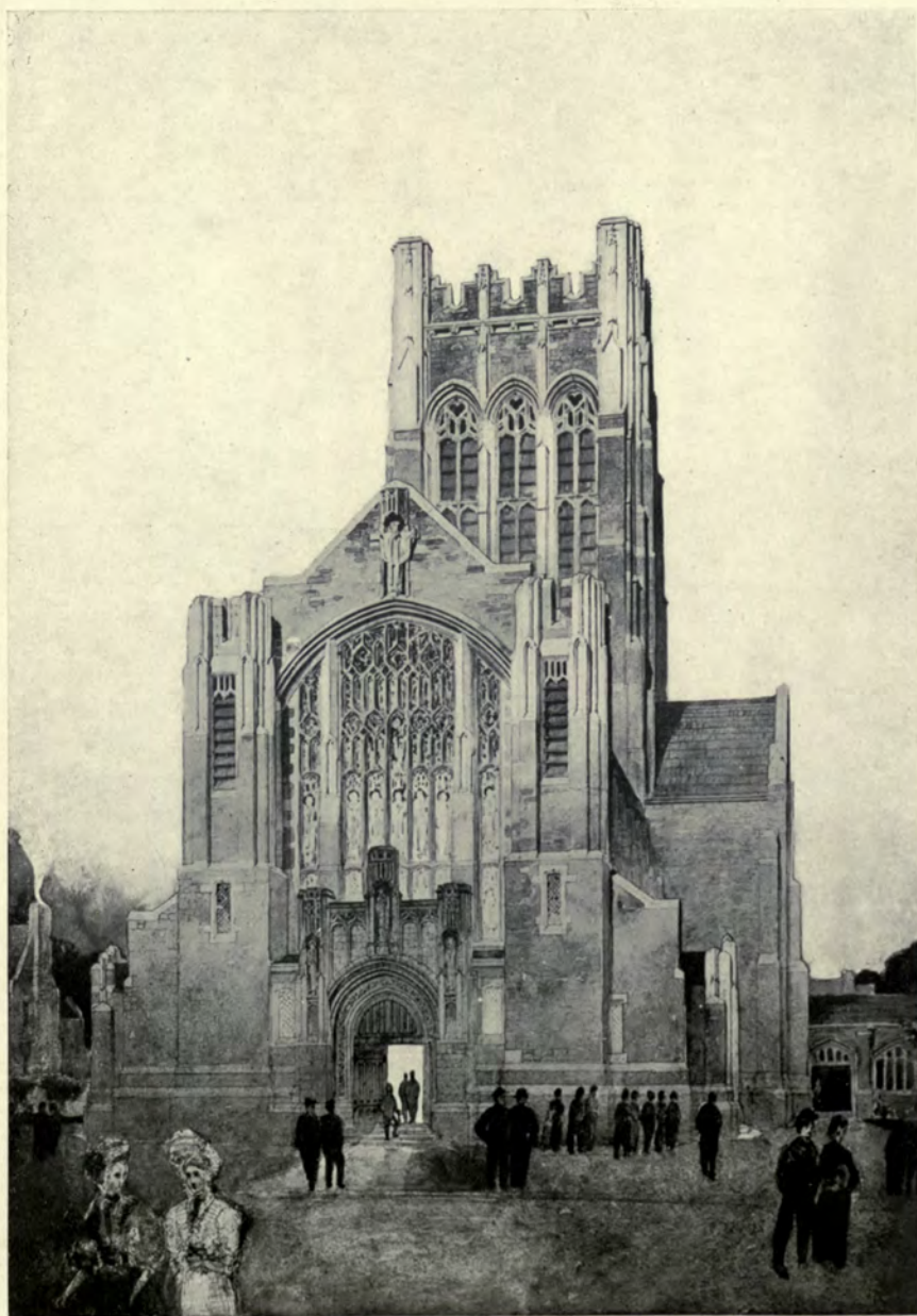
Cathedral, Halifax, Nova Scotia, CRAM, GOODHUE AND FERGUSON, Architects.
