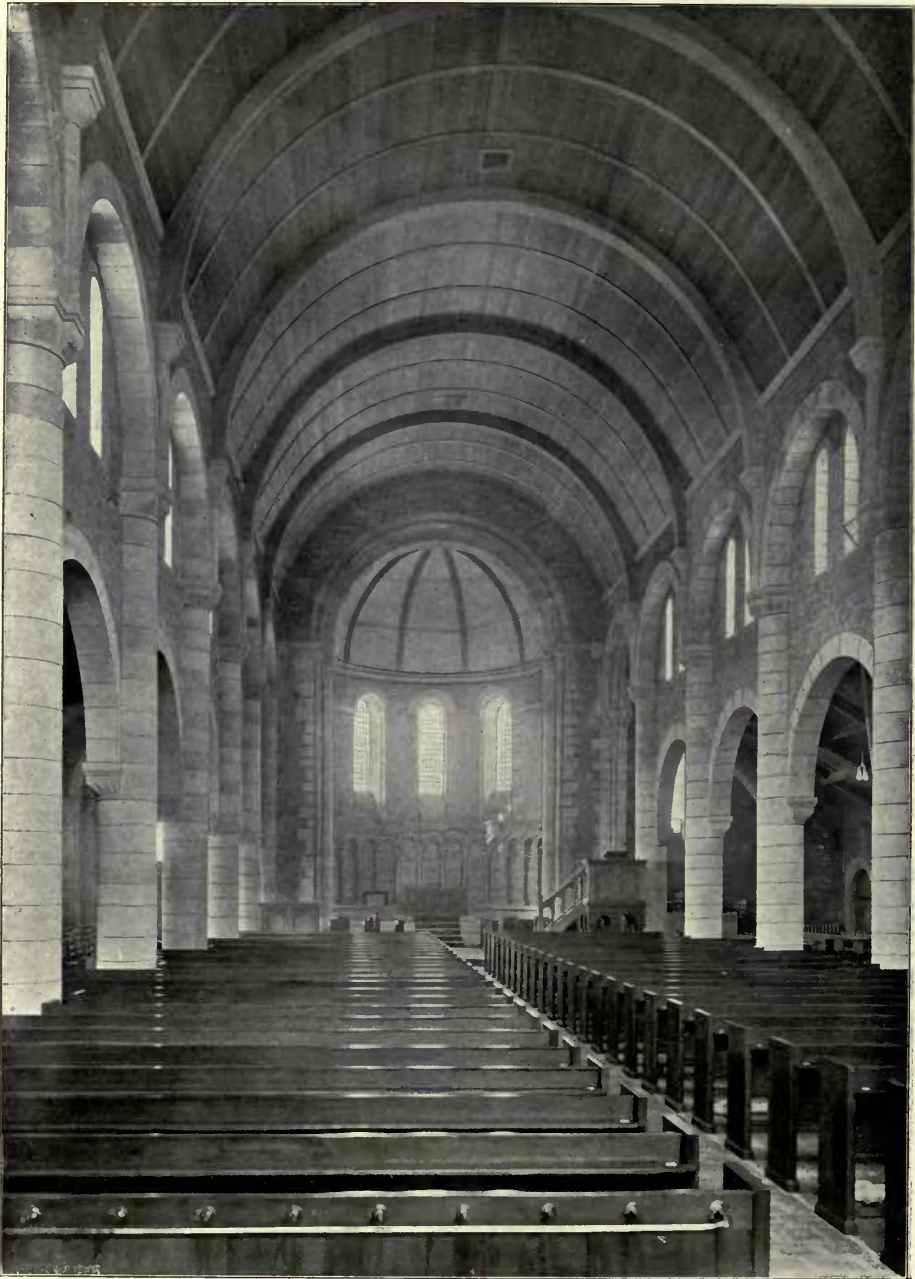
693. St. Luke's Church, Edinburgh, P. MCGREGOR CHALMERS, Architect. Joinery: J. and F. Forrest, Duff Street, Edinburgh.
