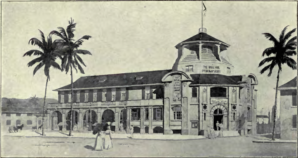
Offices at Jamaica for the Royal Steam Packet Co., LIONEL U. GRACE, Architect. (For Plans, see p. 141.)
