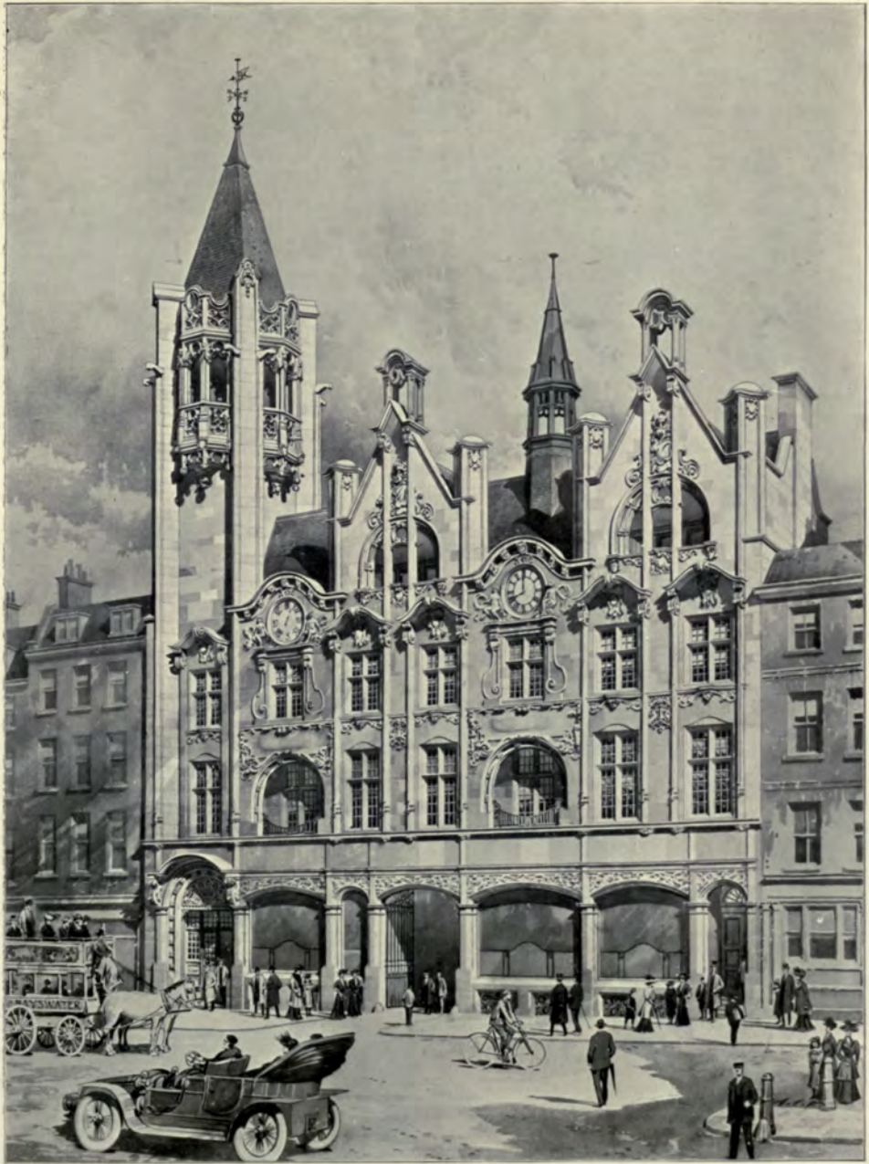
Additions to Messrs. Buchanan's Premises, Holborn, W.C., TREADWELL AND MARTIN, Architects. Contractor: F. G. Minter, Ferry Works, High Street, Putney, S.W. Constructional Steelwork and Fire Resisting Floors on the "Smith Walker" System by: Smith Walker and Co., 11 Tothill Street, Westminster, S.W. The Purbeck-Portland Stone Front up to First Floor level by: The Purbeck Portland Stone Co., Ltd., 11 Tothill Street, Westminster, S.W.
