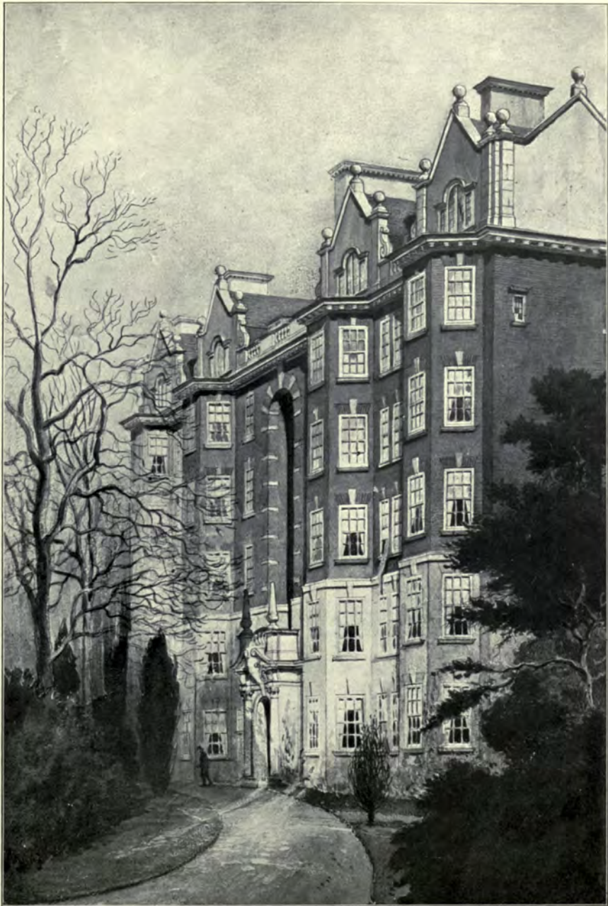
1573. The Pryors, Hampstead, HART AND WATERHOUSE, Architects. Contractor; L. E. Hookway, Beauford Mansions, Beauford Street, Chelsea.
