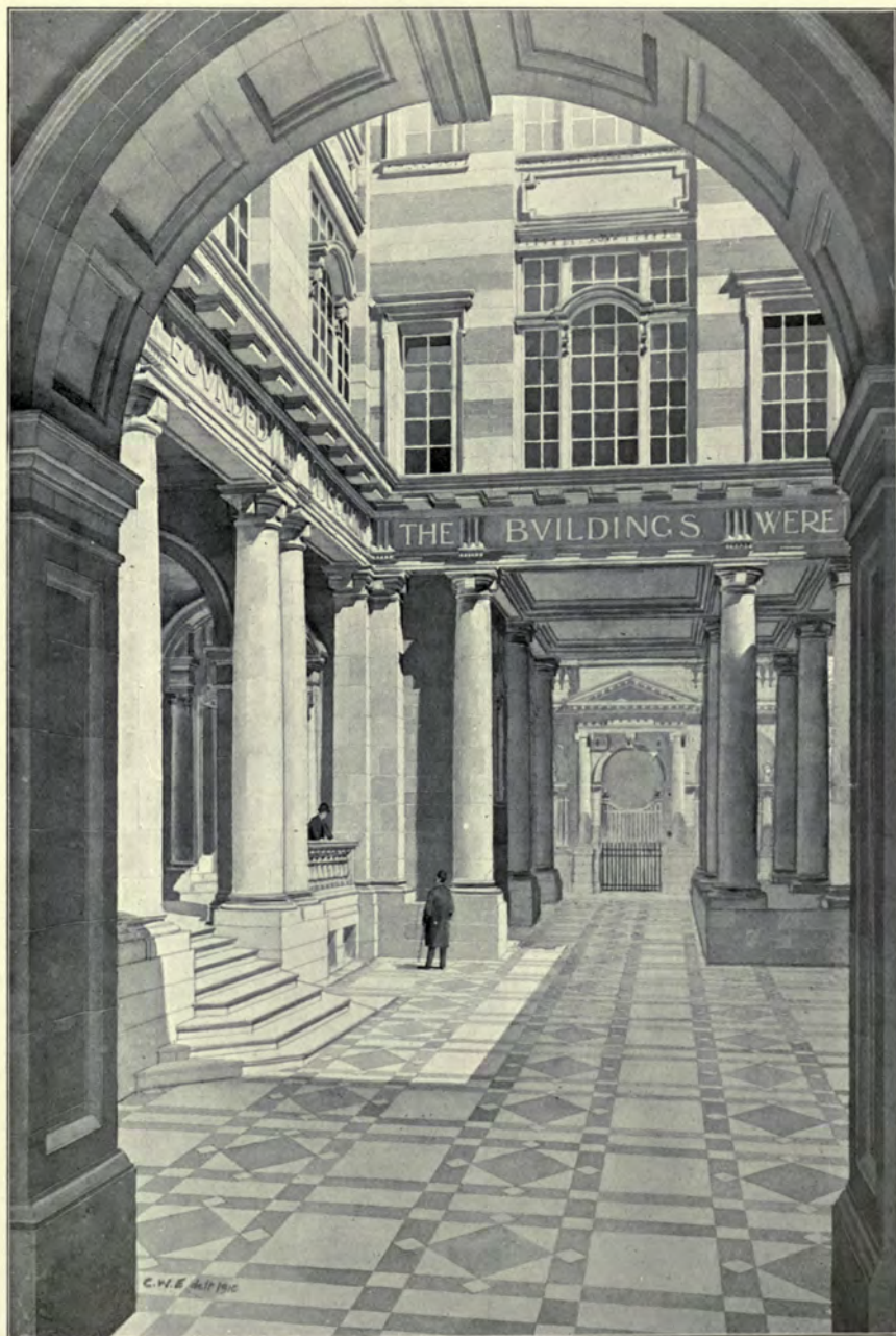
1421. Refuge Assurance Co., Manchester: The Courtyard , PAUL WATERHOUSE, Architect. Eggshell Glazed Terra Cotta: Alfred Whitehead, 35 and 36 Prudential Buildings, Park Row, Leeds.
