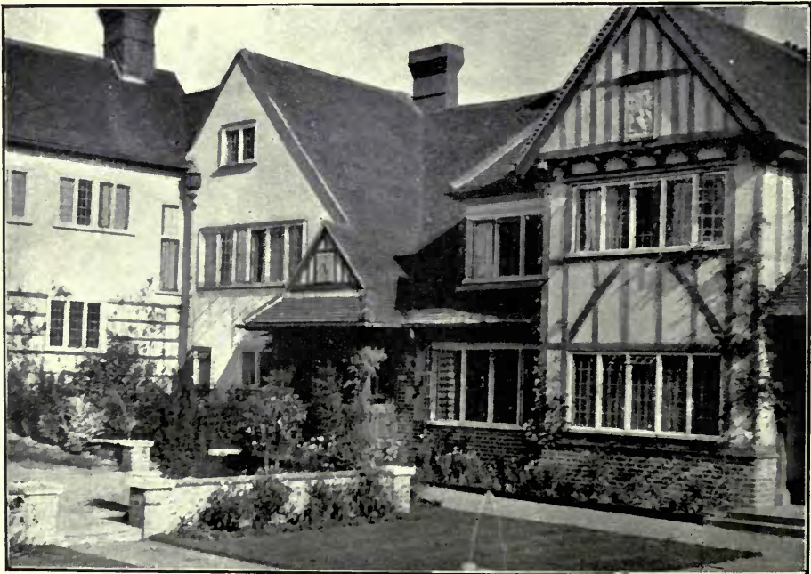
Davenies, Beaconsfield, STANLEY HAMP, Architect.
