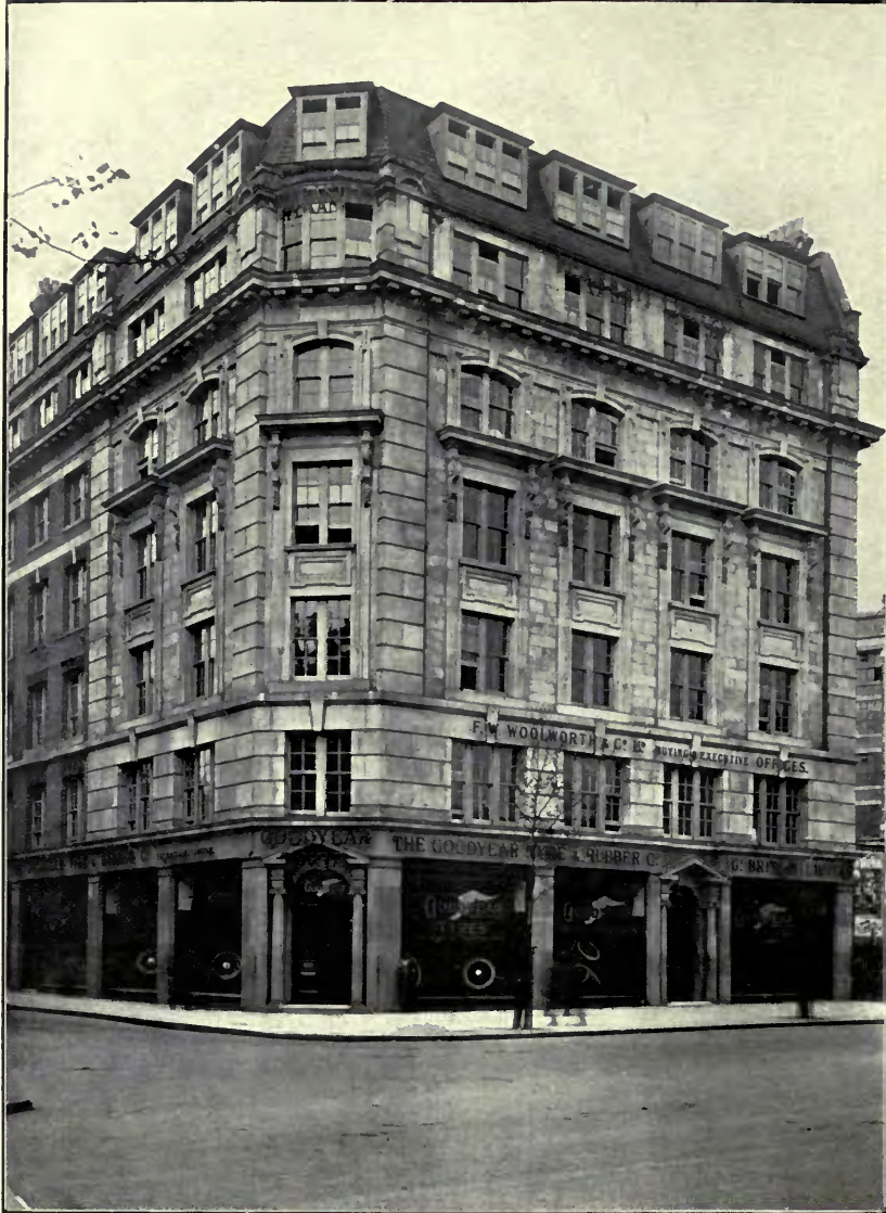
Central House, Kingsway, TREHEARNE & NORMAN, Architects.
