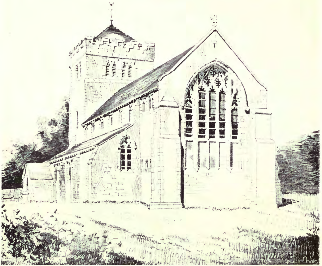
Exterior View of New Church, Carlton-in-Cleveland, Yorks.
