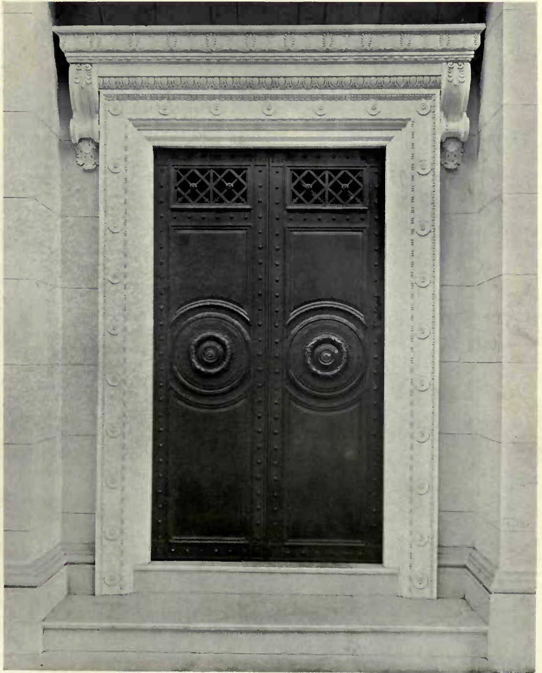
Doorway, Central Heating Pavilion.
