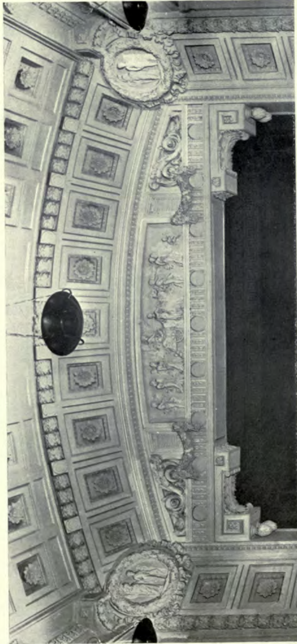
Edinburgh : The New Picture House : Detail of Proscenium Arch. R. ATKINSON & G. L. ALEXANDER, Architects. General Contractors : JAMES MILLAR & SONS, Millar Place, Edinburgh.
