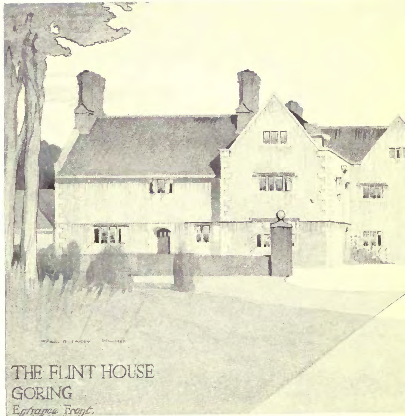
The Flint House, Goring: Entrance Front.
