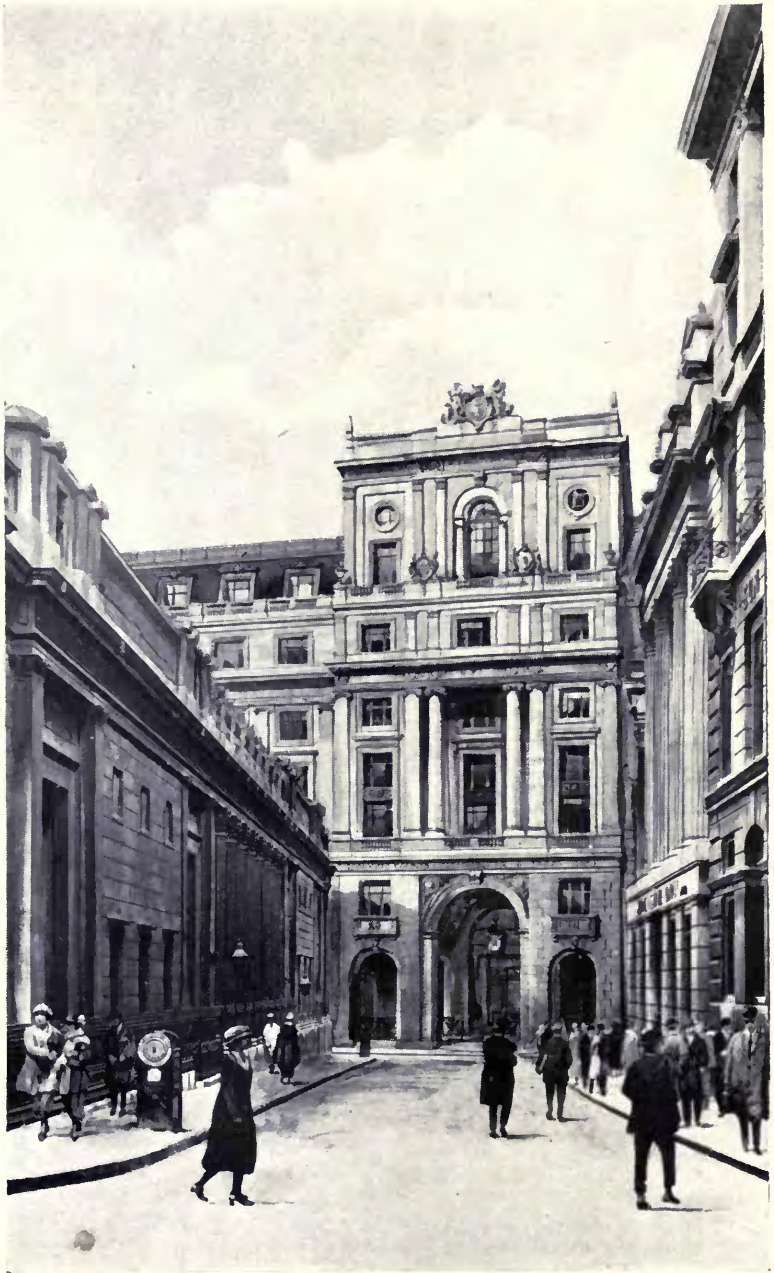
London County Westminster and Parr's Bank, Ltd. Head Office, Lothbury, E.C.
