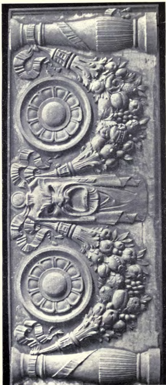
Decorative Panel: Main Entrance.
