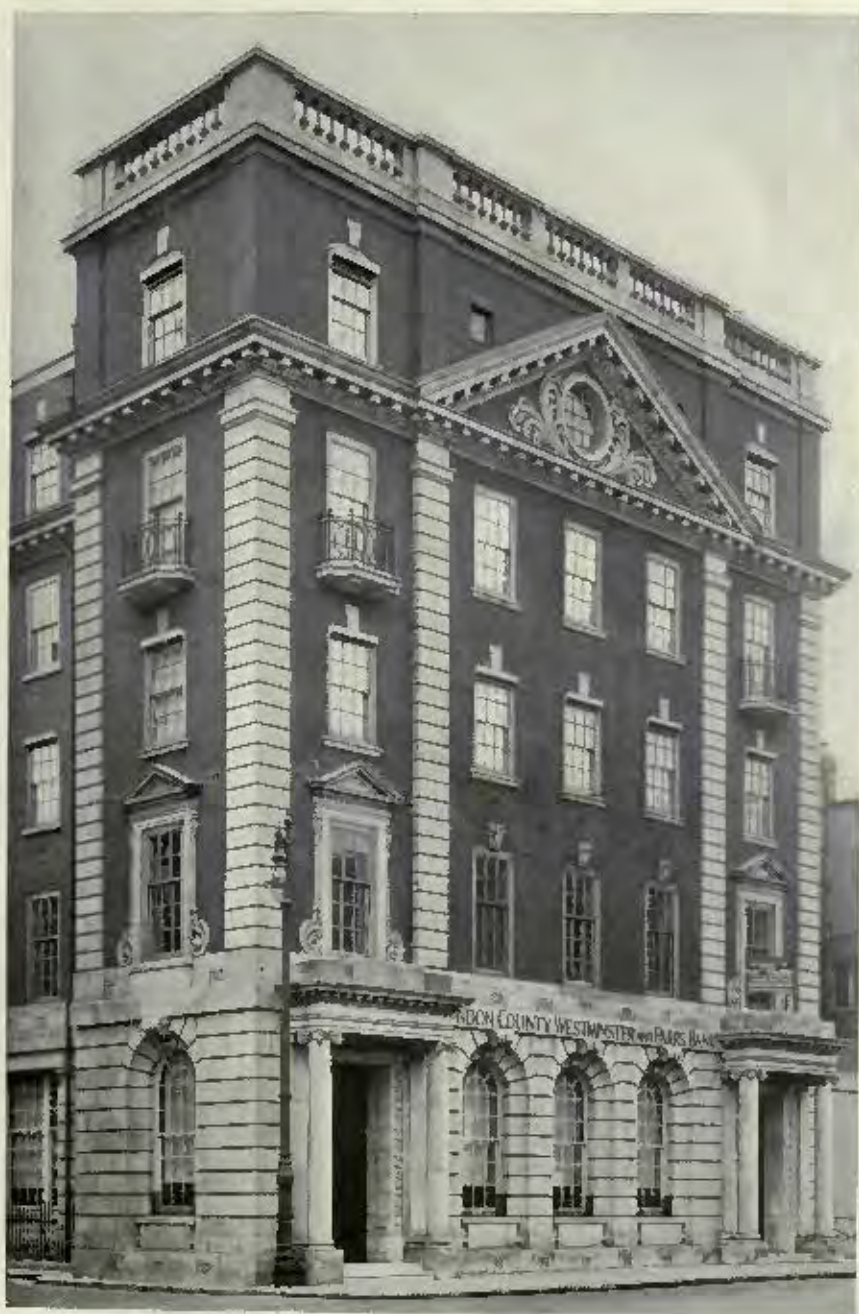
MAYFAIR HOUSE, CARLOS PLACE, GROSVENOR SQUARE, W. EDMUND WIMMERIS AND SIMPSON, ARCHITECTS.
