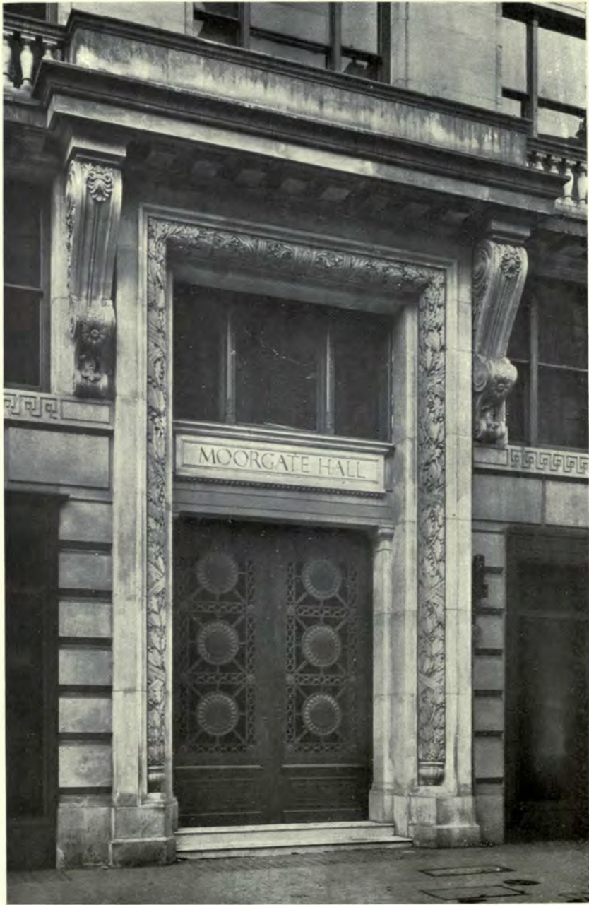
MOORGATE HALL, MAIN ENTRANCE : DETAIL.
