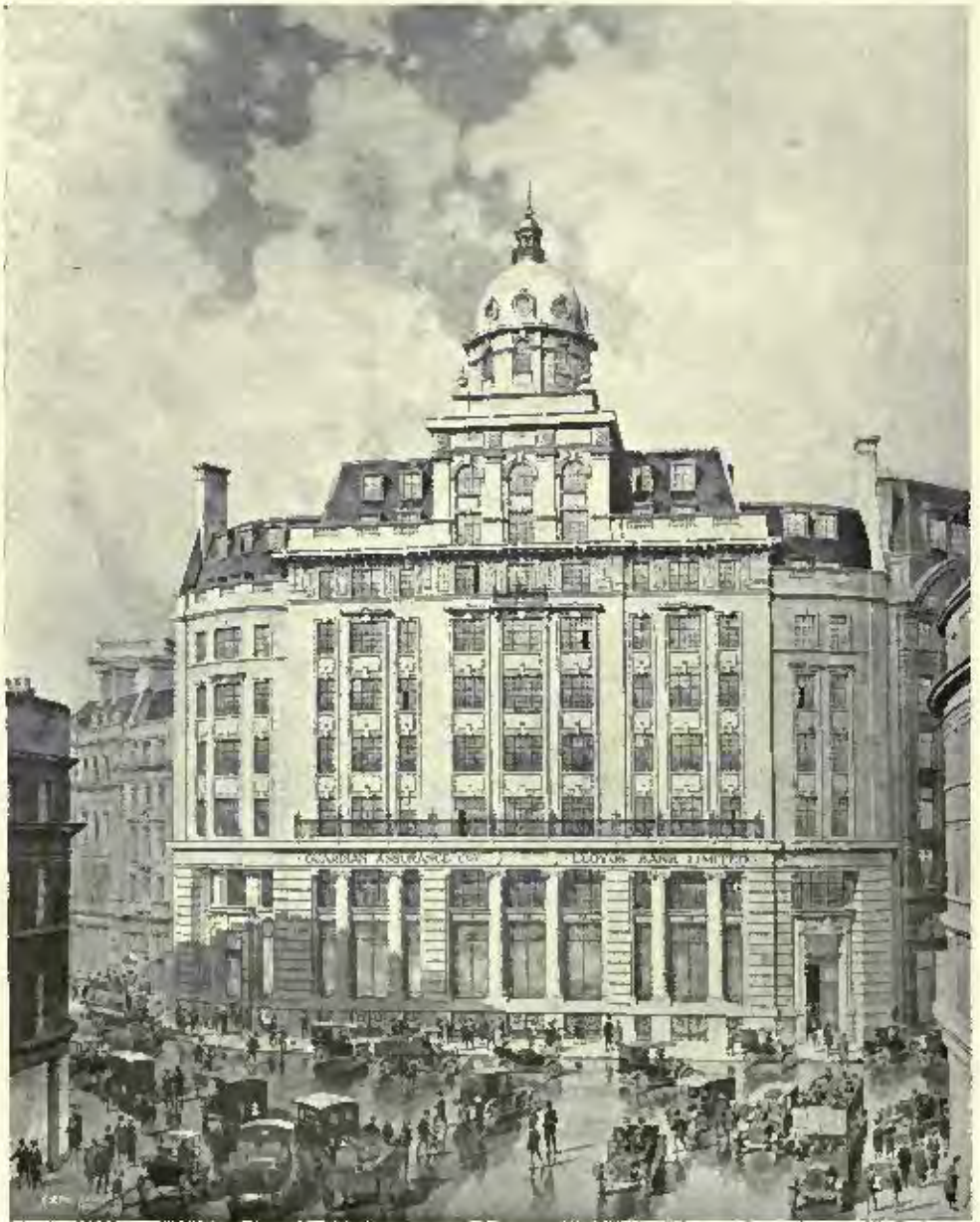
NEW PREMISES, KING WILLIAM STREET.
