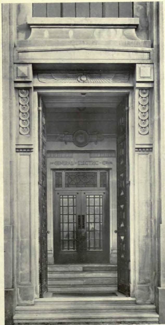
GENERAL ELECTRIC CO., WITTON, BIRMINGHAM. ADMINISTRATION OFFICES : MAIN ENTRANCE. WALLIS, GILBERT AND PARTNERS, ARCHITECTS.
