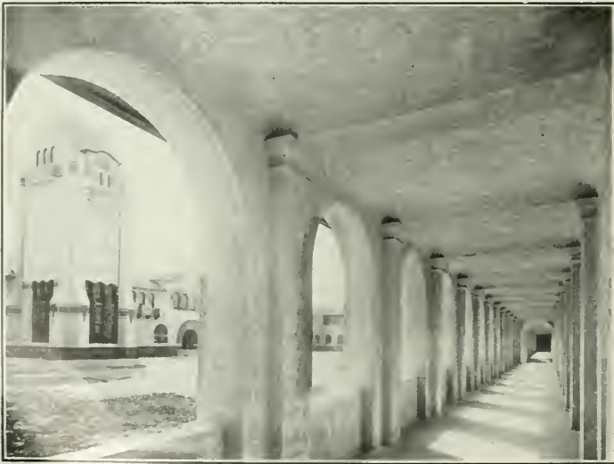
Looking Southeast Toward the Tower, from Arcade
