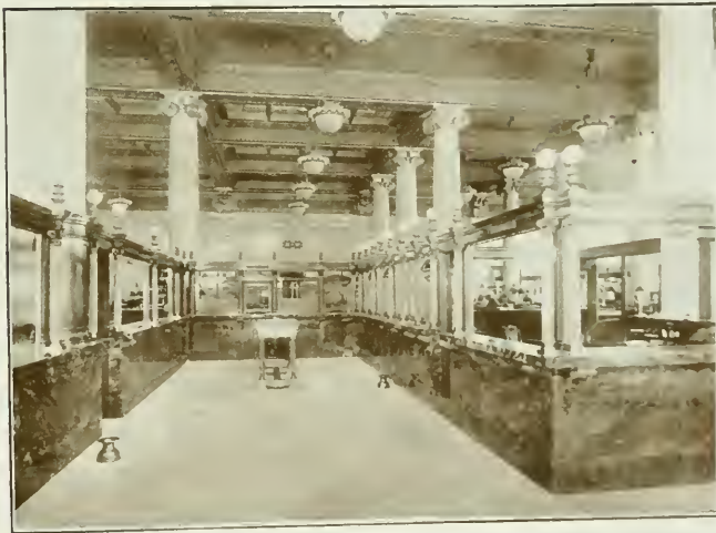
Interior, Security Savings Bank
