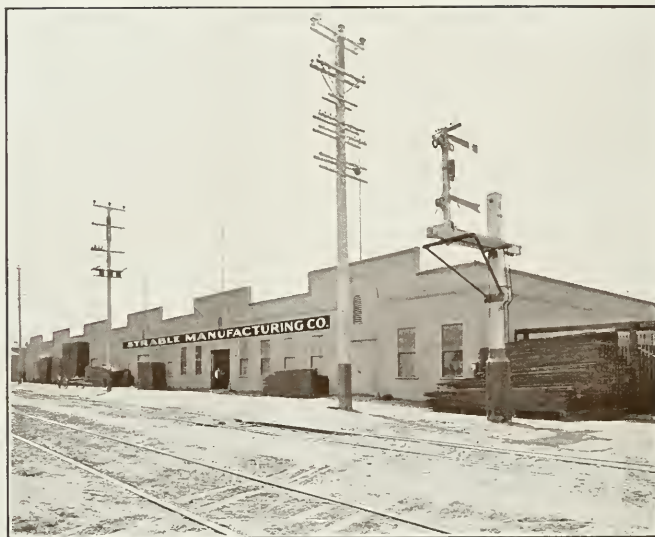
Pacific Coast Warehouse of Strable Manufacturing Company
