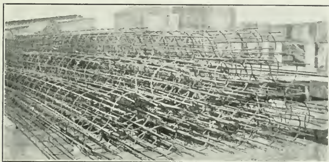
Cage-like Device of Reinforcing Bars and Bands for Concrete Piles
