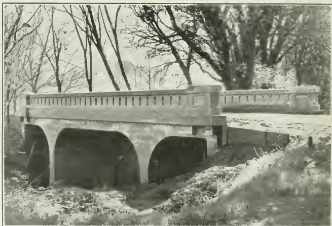
Fig. 5—Reinforced Concrete Flat Slab Bridge, City of Ross, Marin County, California John B. Leonard, Engineer
