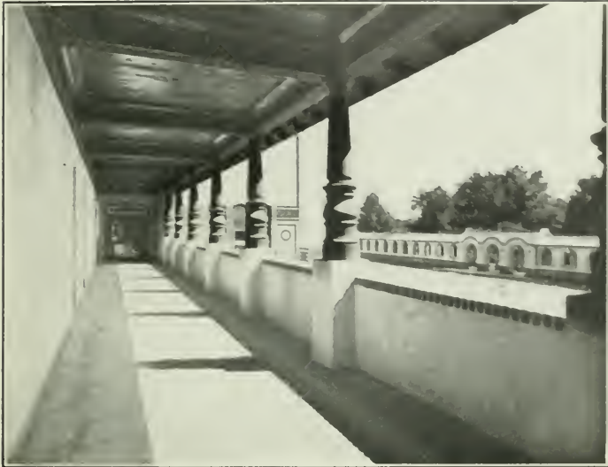
Looking West from Second Story Open Corridor
