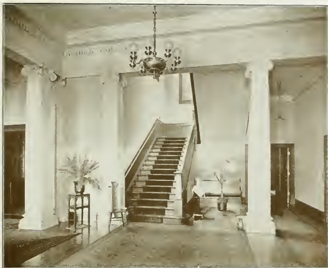
Interior, Bresee Bros. Building
