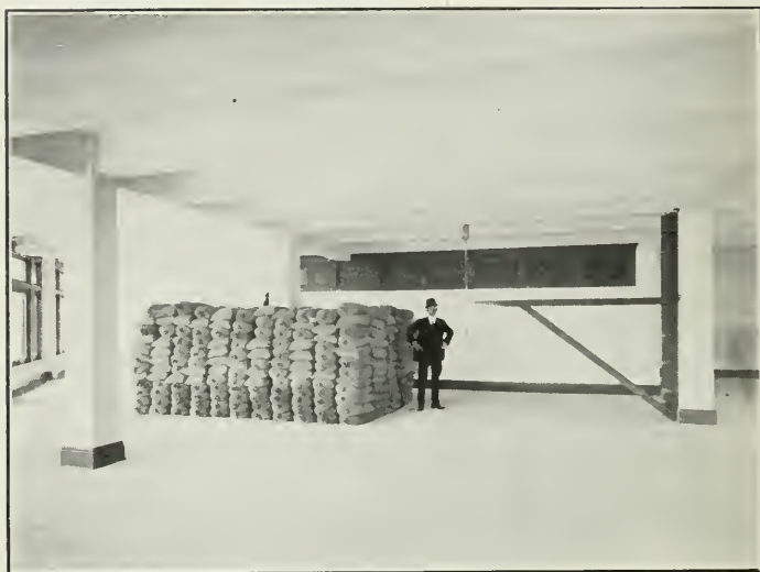
MacDonough Building, San Francisco, Showing Floor Tests MacDonald & Applegarth, Architects
