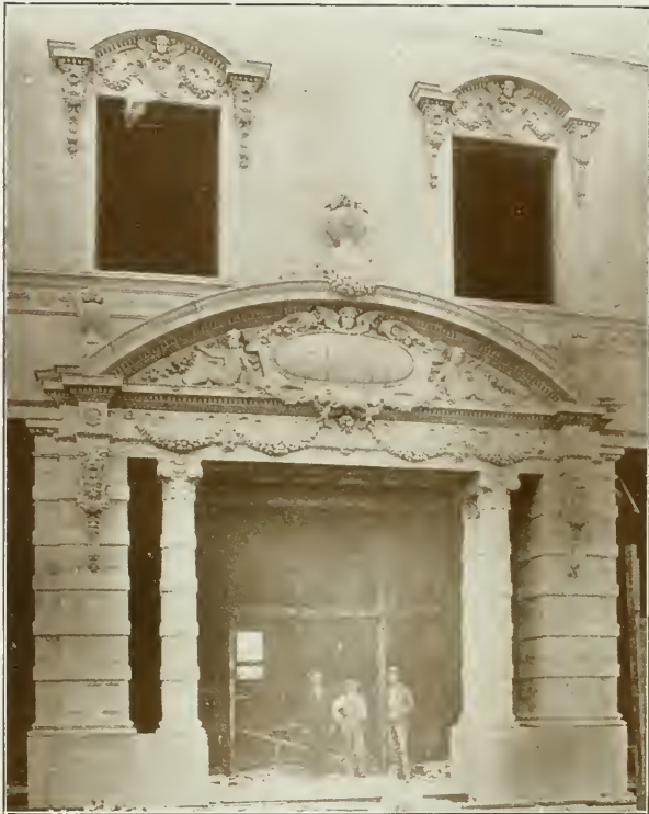
Detail of Entrance, Angelus Hotel
