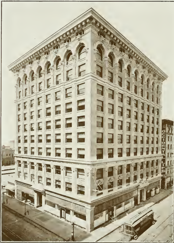
Central Building, Los Angeles Parkinson & Bergstrom, Architects
