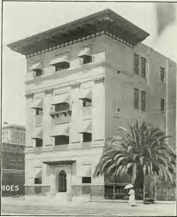
Pacific States Telephone Building, San Jose
