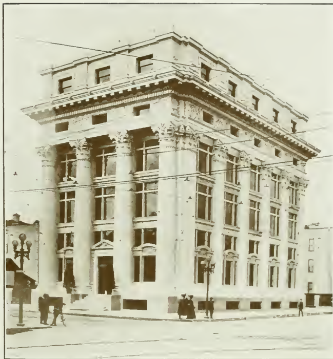
Pacific Mutual Life Insurance Building, Los Angeles, Parkinson & Bergstrom Architects
