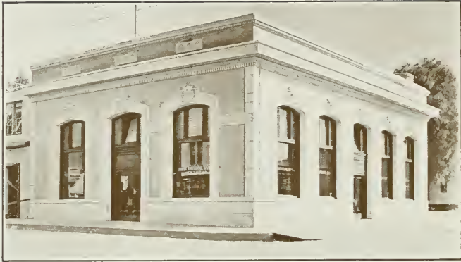
First National Bank Building, Monrovia, Cal. Parkinson & Bergstrom, Architects
