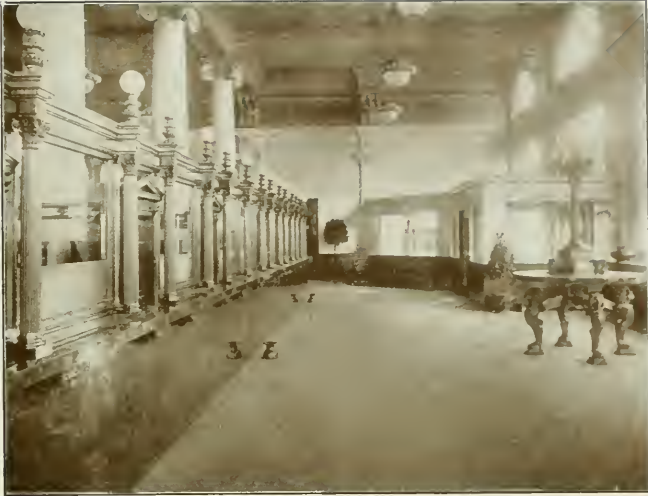
Interior, Security Savings Bank
