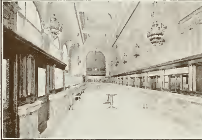
Interior of Banking Room, London Paris National Bank, San Francisco Albert Pissis, Architect
