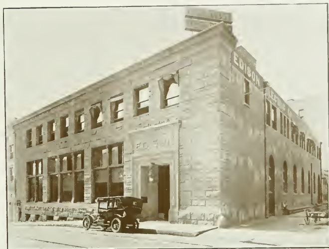
Edison Electric Building, Los Angeles
