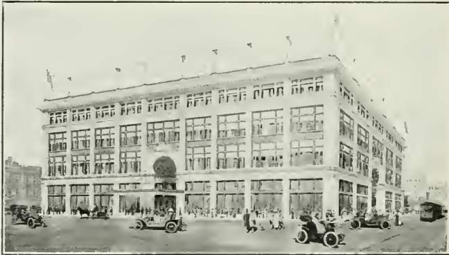
Capwell Department Store Building, Oakland C. W. Dickey, Architect
