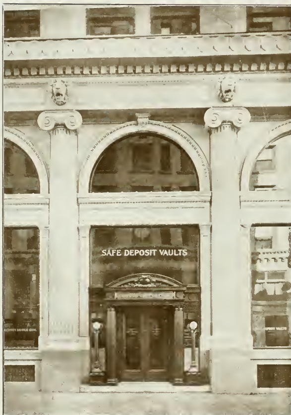
Detail of Entrance, Security Savings Bank
