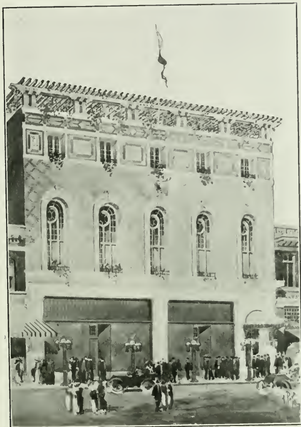
Elks' Building, Marysville, California Walter H. Parker, Architect
