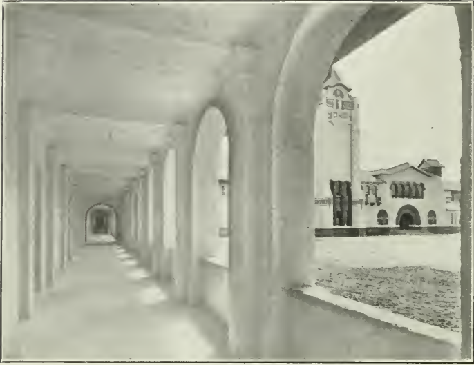
Arcade, Showing Massive Concrete Arches
