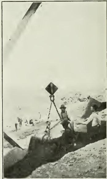
Derrick at Work in the Ione Sandstone Quarries
